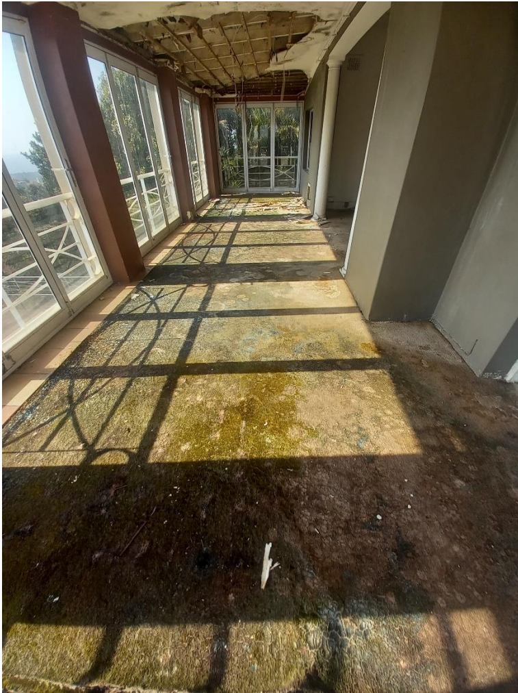
FIG. 8. View of existing balcony
