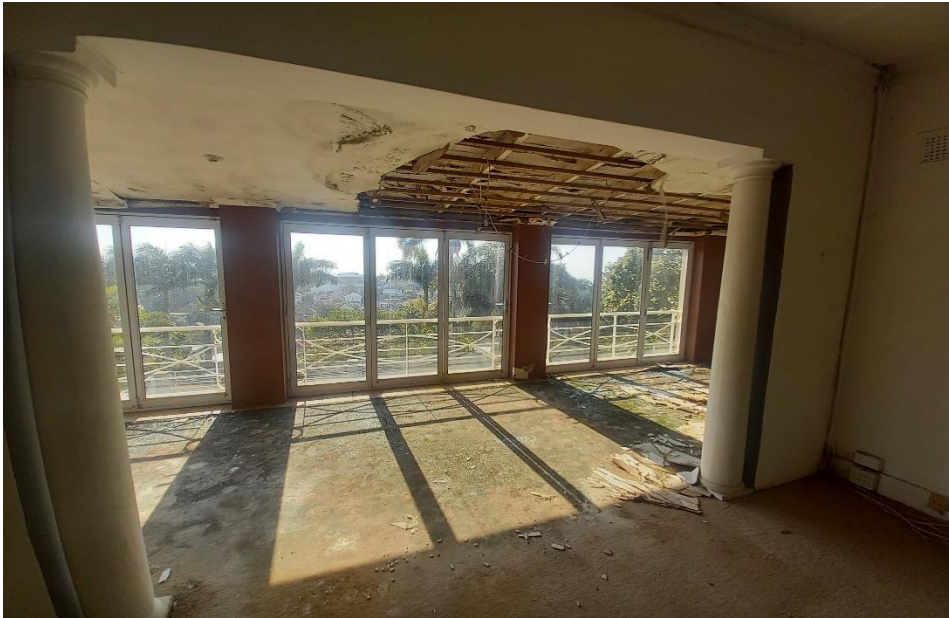
FIG. 7. View from master bedroom to existing balcony
