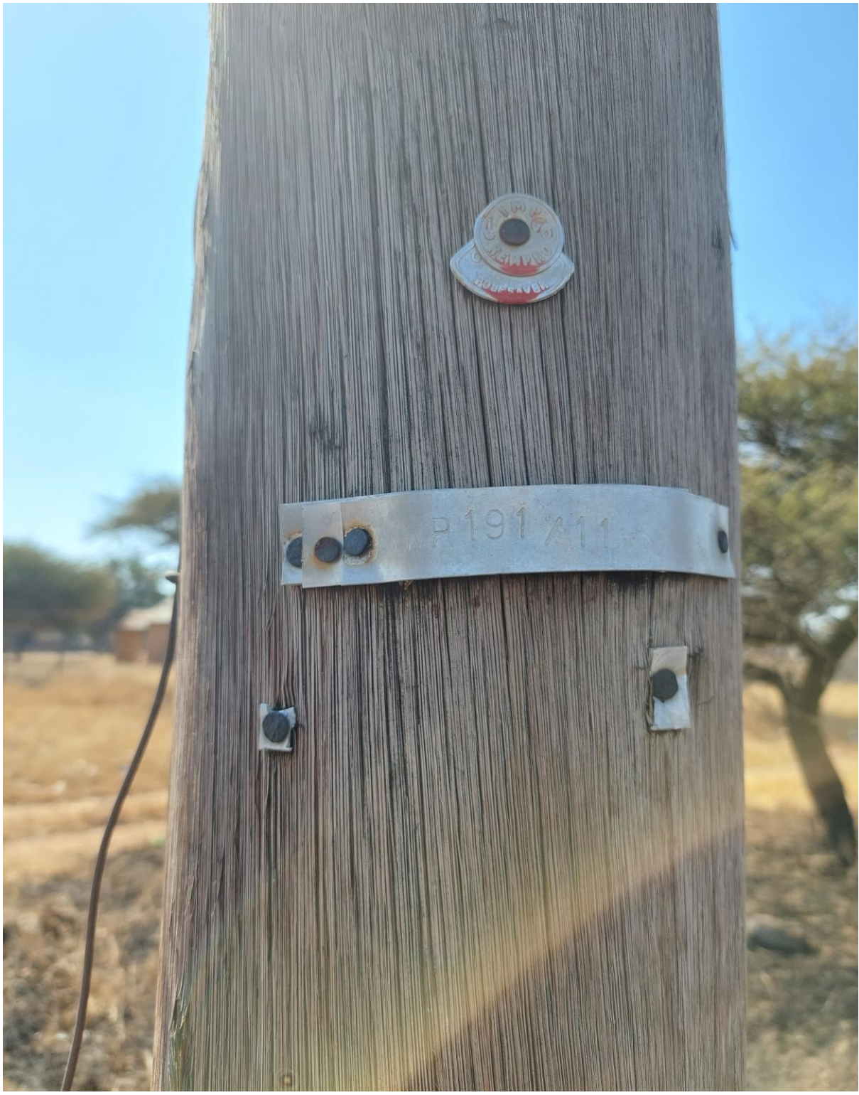
PICTURE SHOWING THE POLE NUMBER WHERE THE PROPOSED LINE WILL BE CONNECTED
