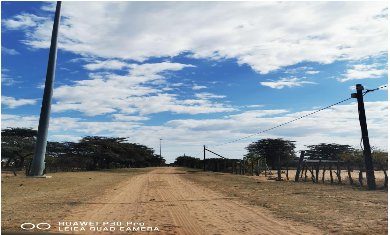
Figure 3: Existing road and Powerline
