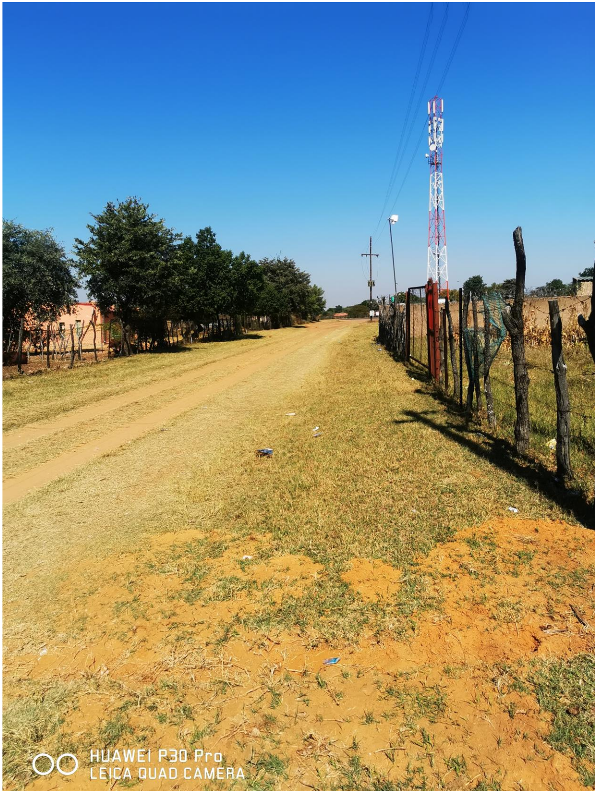
Figure 4: Picture showing road, fence and houses infrastructure in the project area
