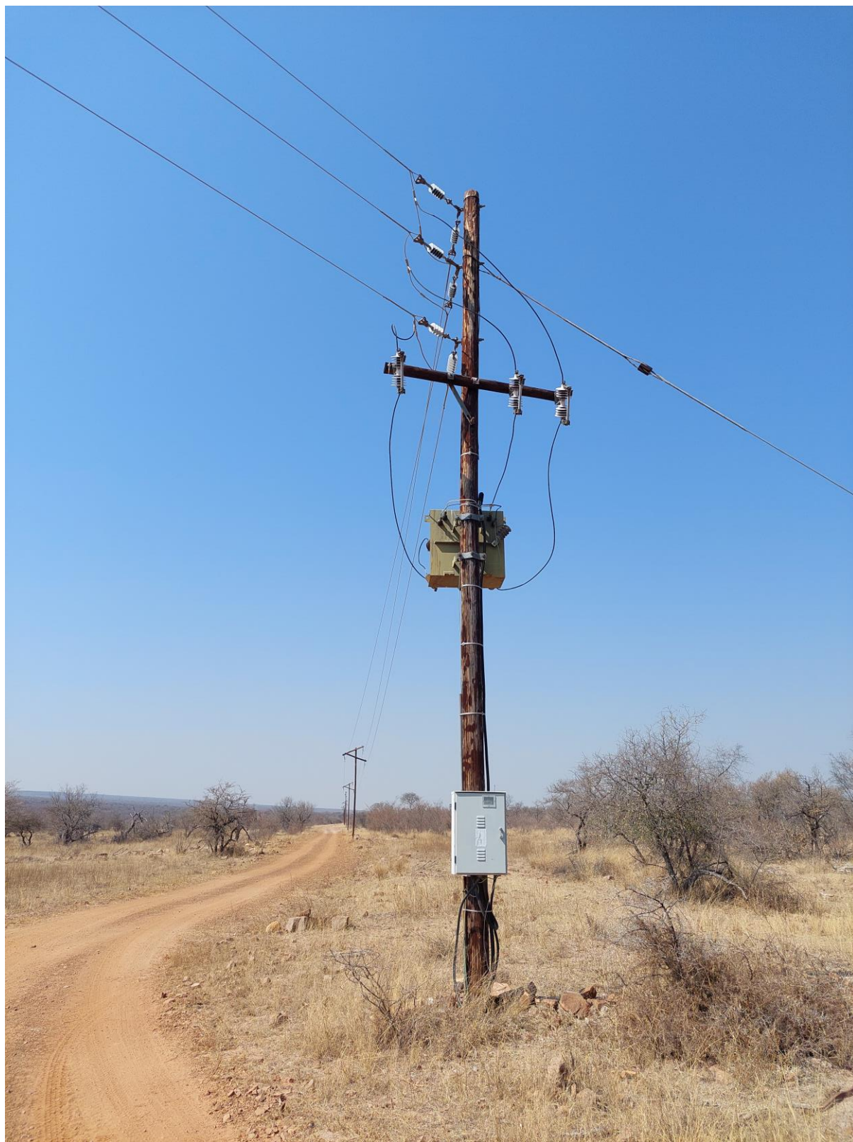
PICTURE SHOWING THE EXISTING POWERLINE IN THE SYUDY AREA
