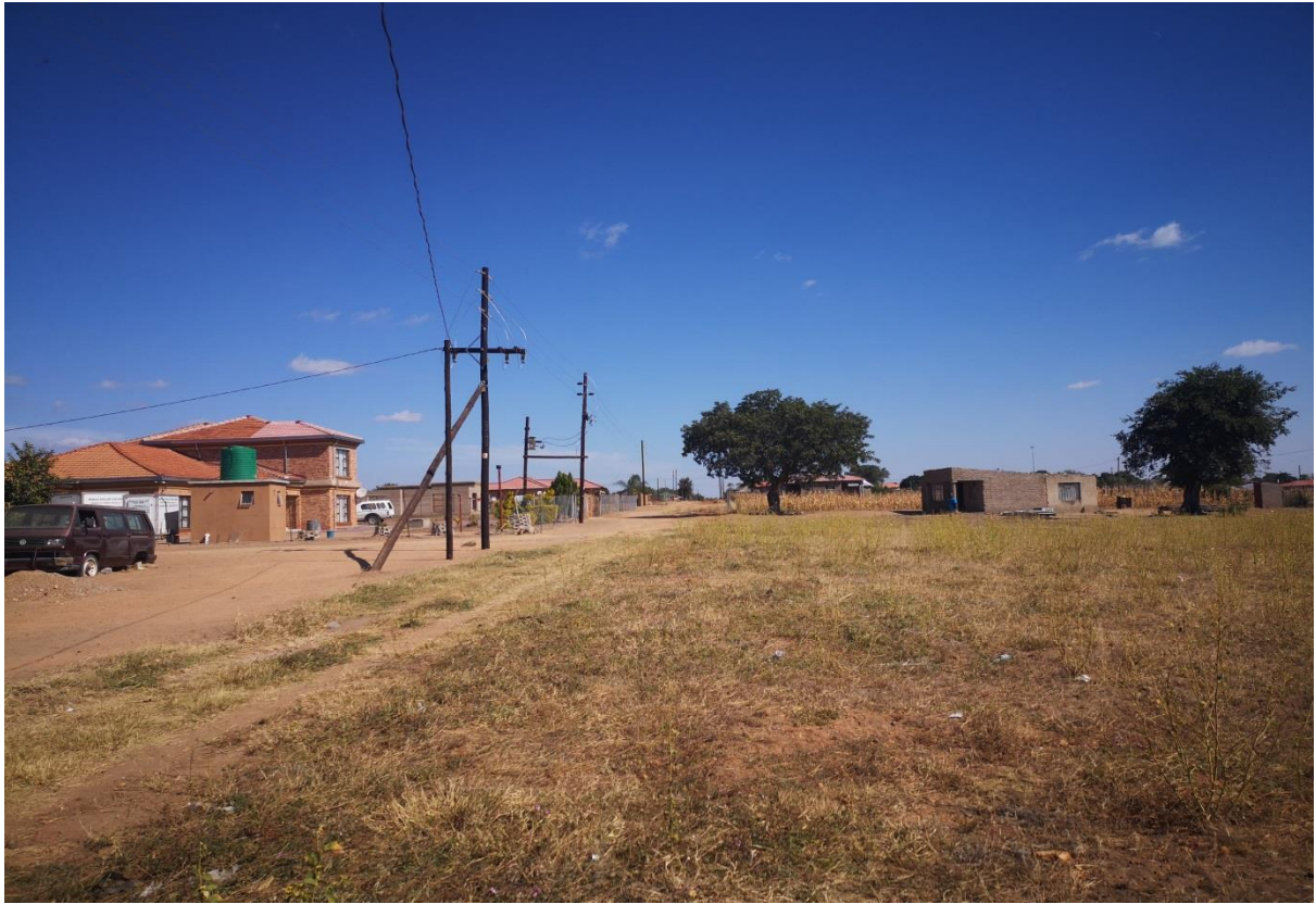
Picture 3: Existing powerlines and the surrounding
