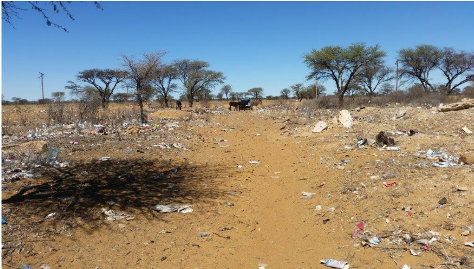
Plate 1.1: Interior view of the Piet Plessis landfill, please note donkey feeding on waste in the background, site viewed from the north
