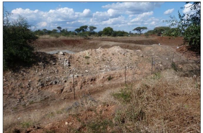
Figure 8 | Extensive earthworks at Open Pit 36W
