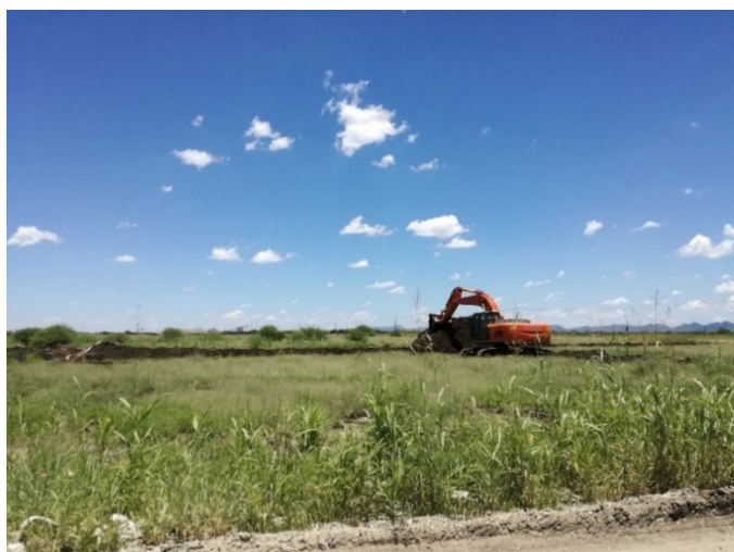
Figure 18 | View from within Pit 62E area, looking west
