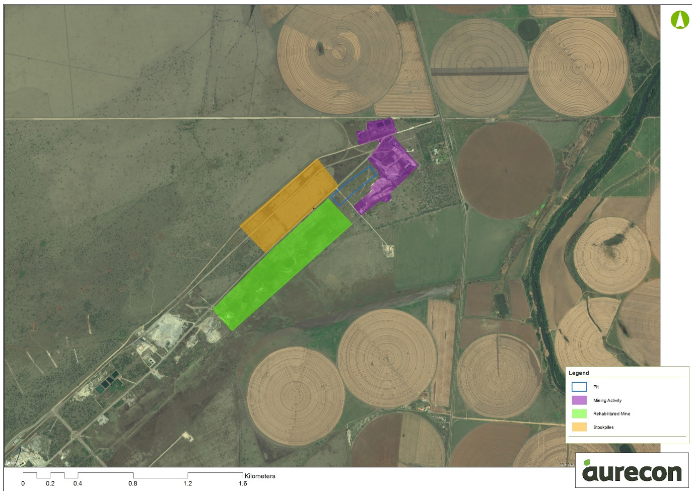
Figure 8 | Map of Pit 62E location, showing its position surrounded by a substantially transformed landscape
