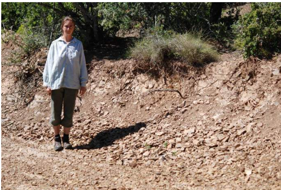
Figure. 17. Small road aggregate quarry in upper Lake Mentz Subgroup shale. Point 7 (fig. 7)
