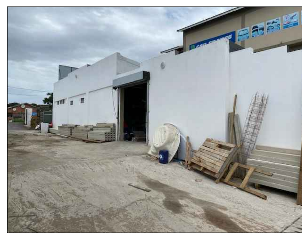
Side View of Ex. Warehouse
