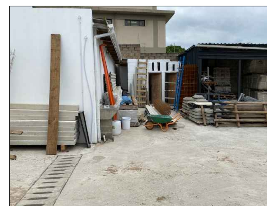
Back Yard with Toilet Outbuilding and part of Awning to store goods
