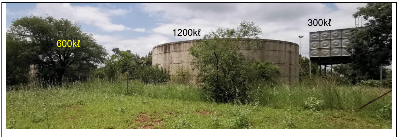
Figure 11 Mtititi / Plange water storage at Altein plant
