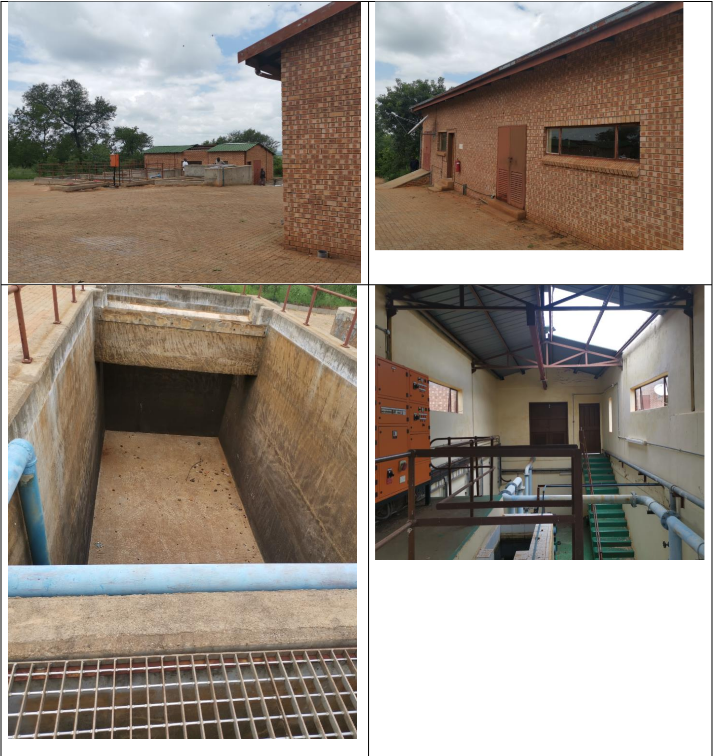
Figure 10 Currently defunct, Altein Water Treatment Works
