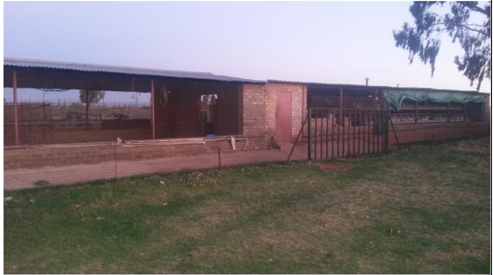
Figure 1 Some of the existing poultry houses
