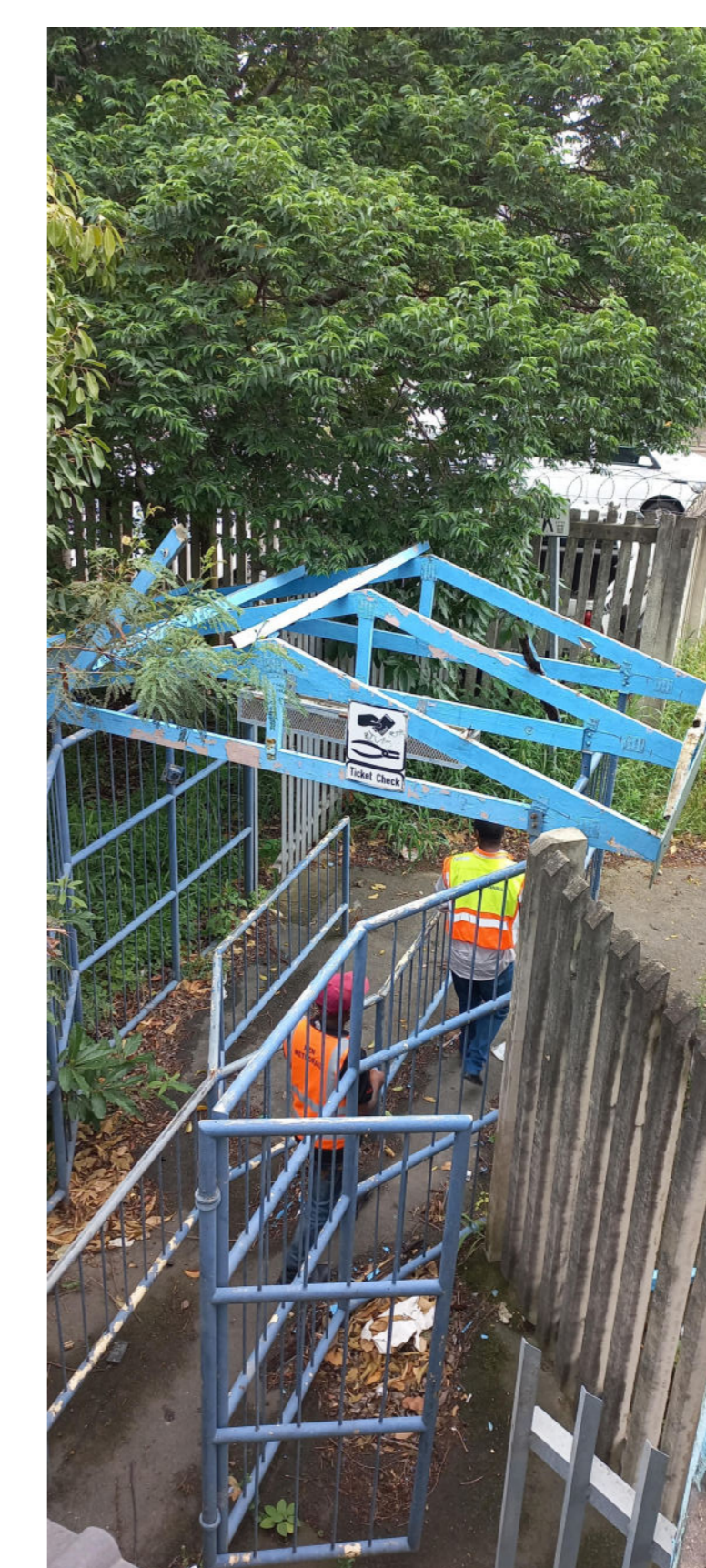
3 - EXISTING ENTRANCE STRUCTURE
