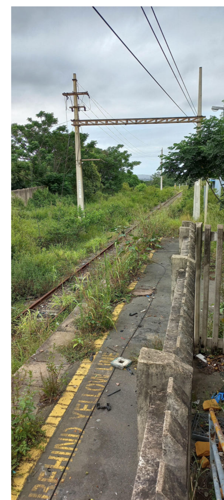
2 - EXISTING STATION PLATFORM
