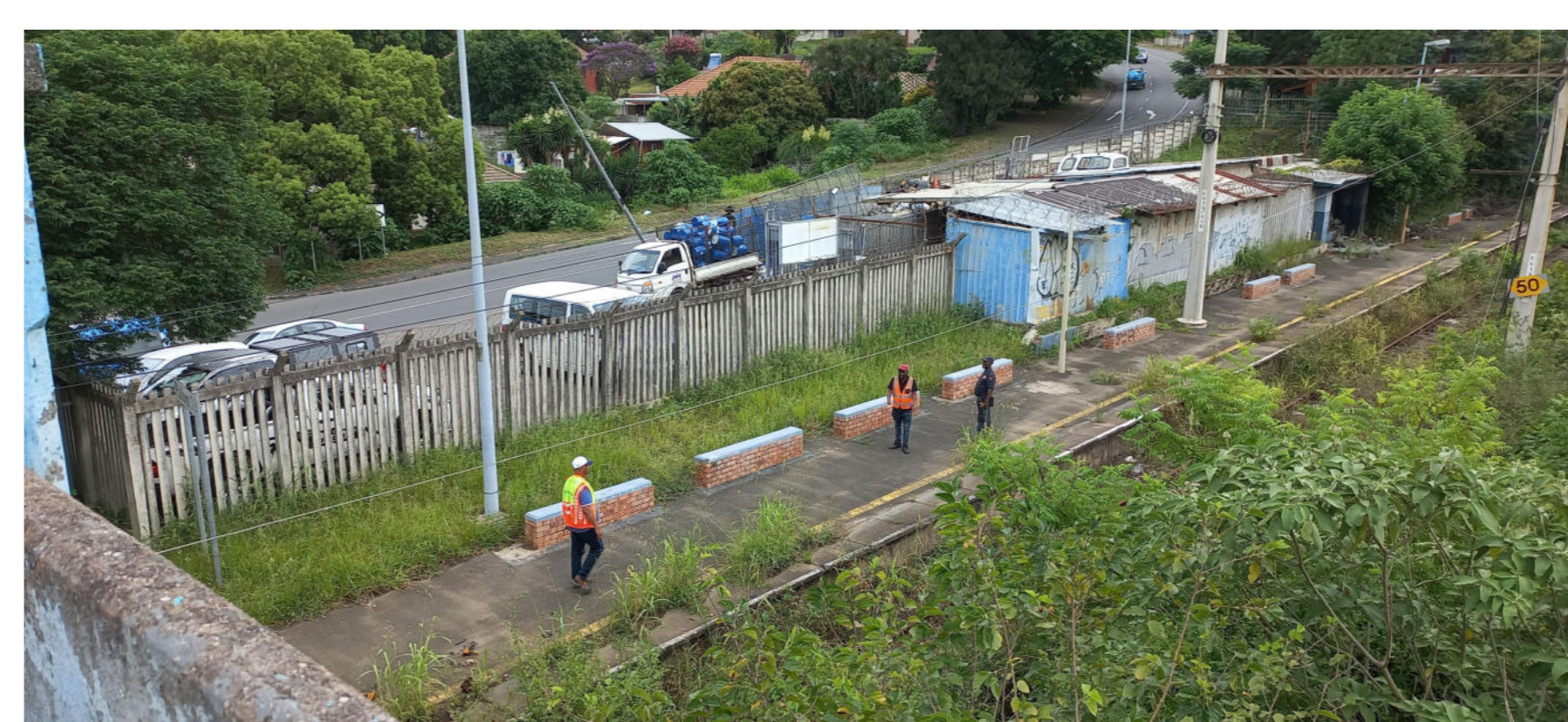
6 - EXISTING PUBLIC SEATING (UNLAWFUL WORK)
