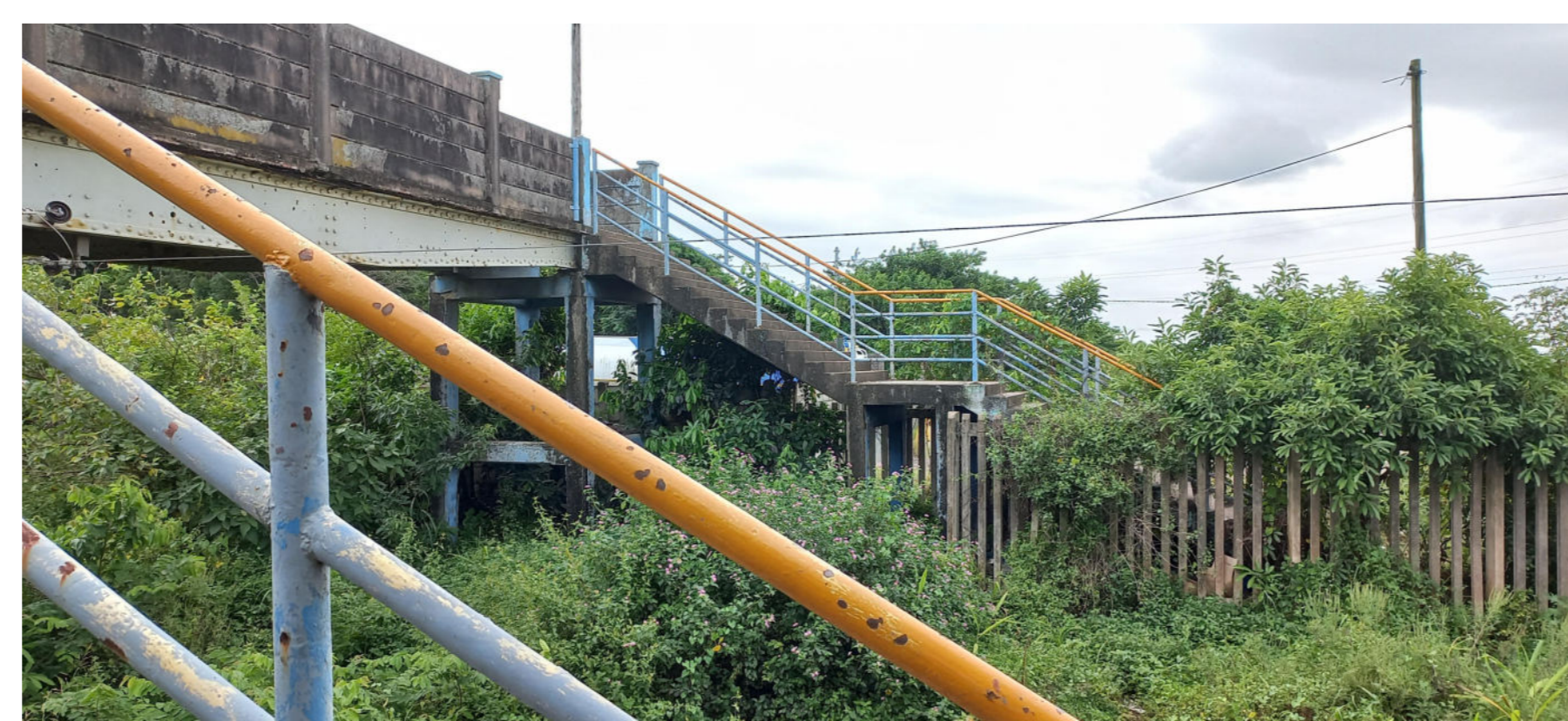
5 - EXISTING PEDESTRIAN BRIDGE
