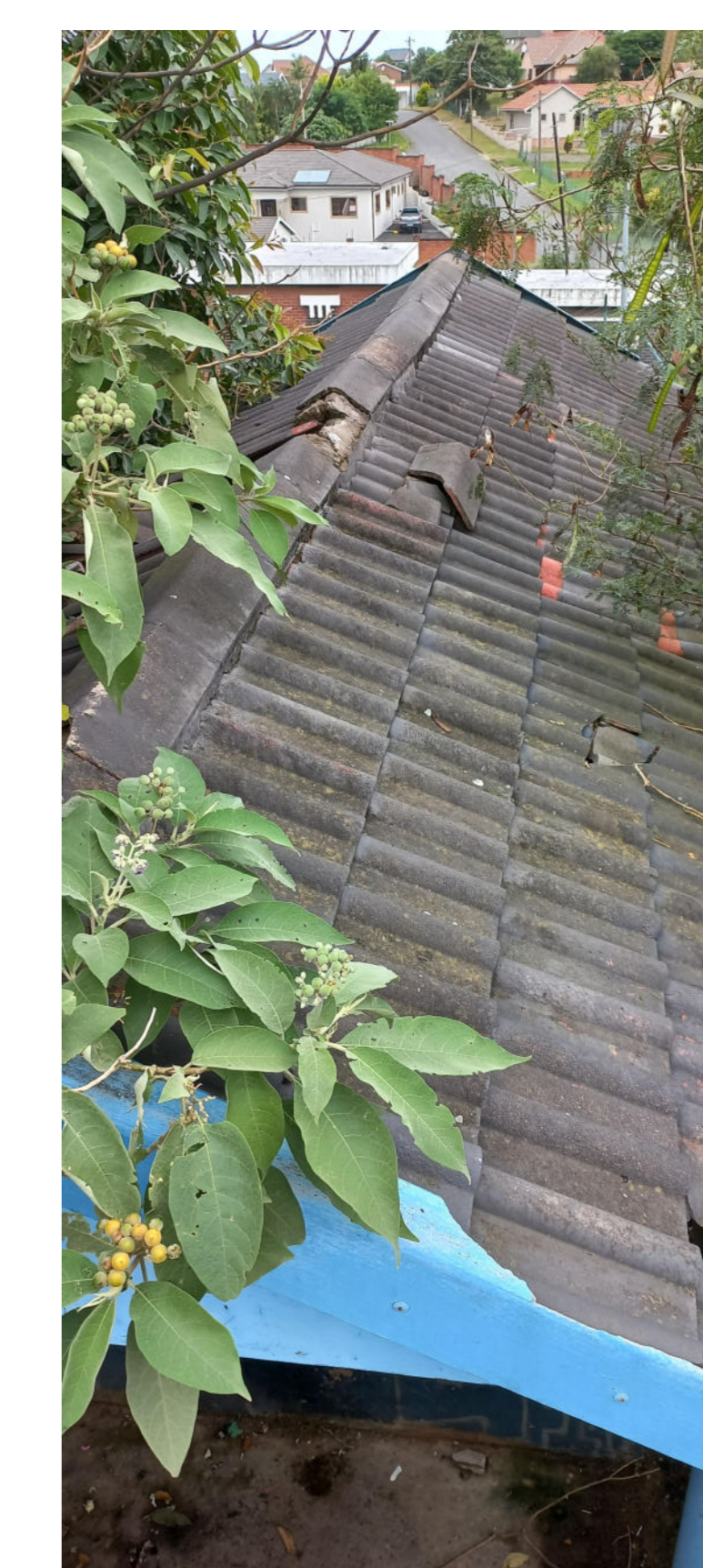
4 - EXISTING TICKET OFFICE
