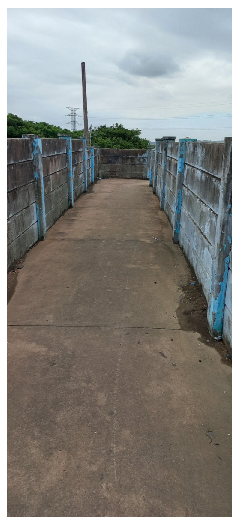
1 - EXISTING PEDESTRIAN BRIDGE
