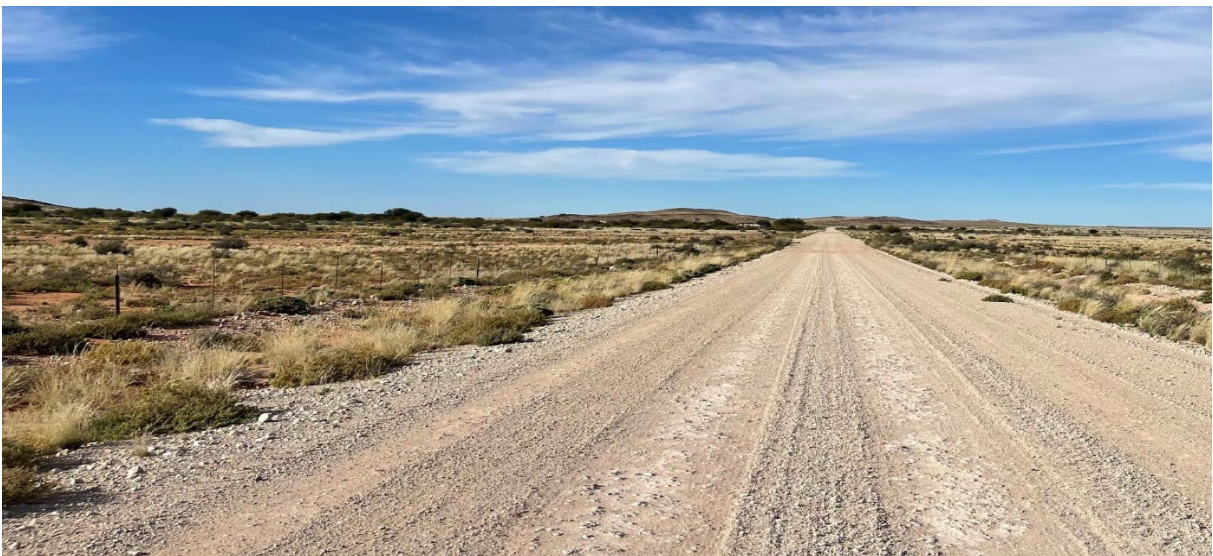
Figure 7.10 Existing Road DR2986 @ Km 153.99 – West Approaching
