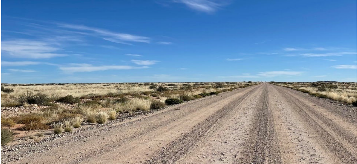
Figure 7.8 Existing Road DR2986 @ Km 153.99 – West Approaching
