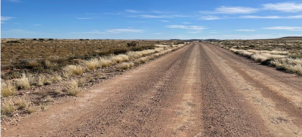
Figure 7.11 Existing Road DR2986 @ Km 148.11 – East Approaching
