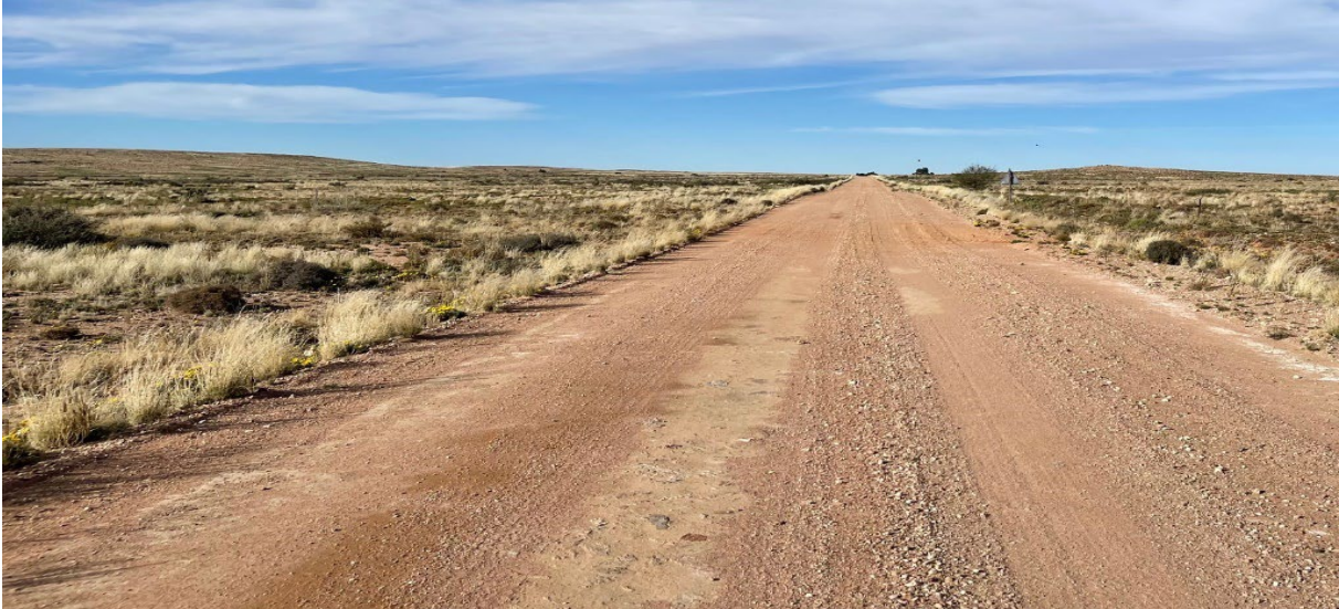
Figure 7.14 Existing Road DR2986 @ Km 148.11 – West Approaching
