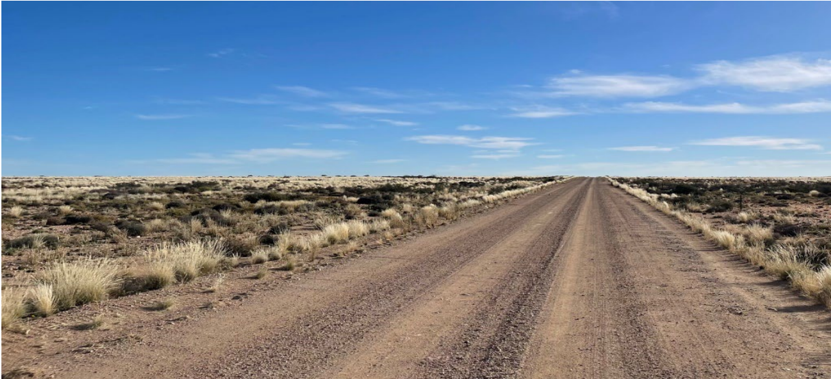
Figure 7.18 Existing Road DR2986 @ Km 142.80 – East Approaching
