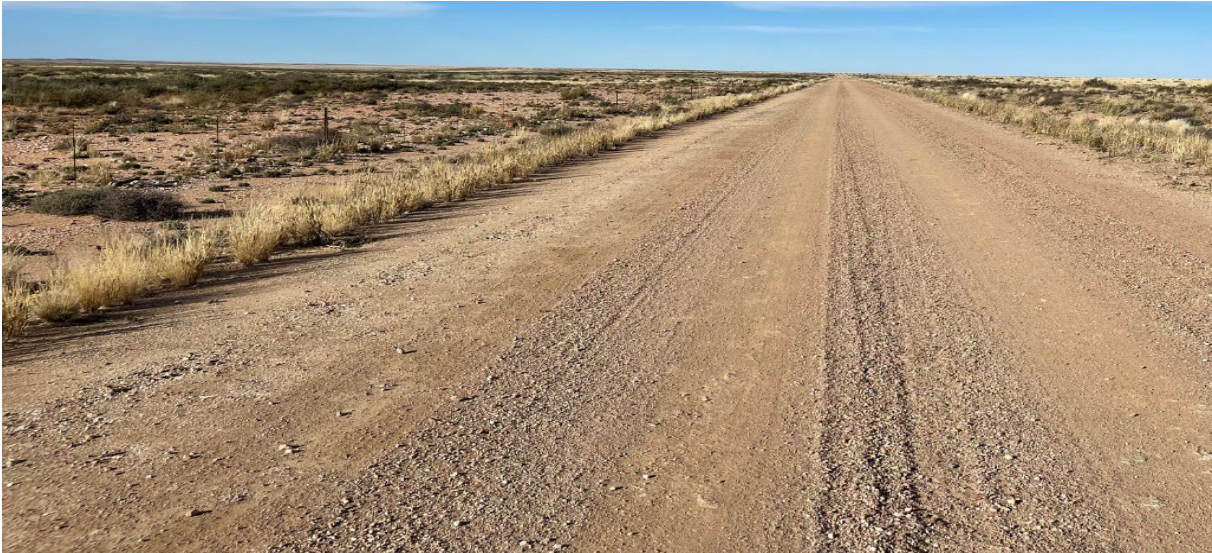
Figure 7.21 Existing Road DR2986 @ Km 142.80 – West Approaching
