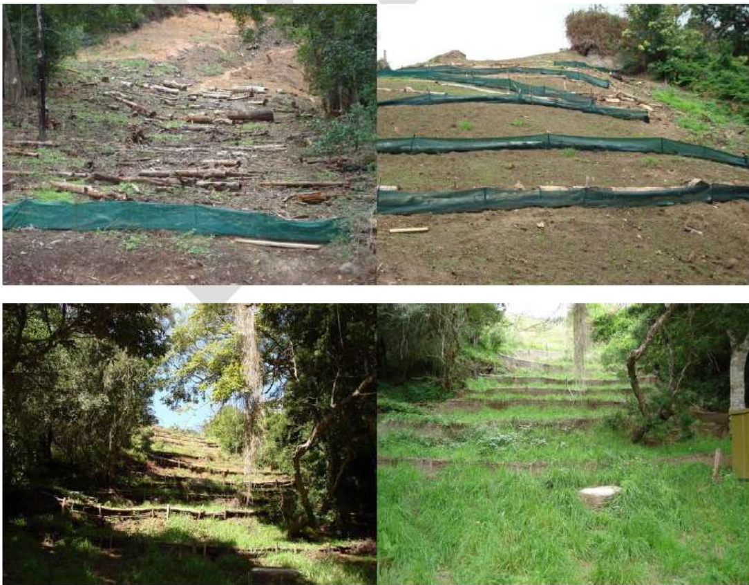
Example of soil erosion protection by means of silt fences and logs
