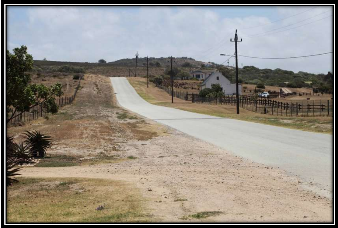
Photograph 7: 4 View of tar road north of the site. (January 2020) Photo: R.F. Terblanche
