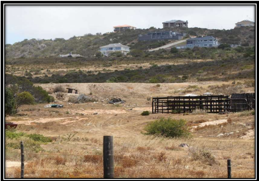
Photograph 6: View towards ground wall of dam (artificial waterbody) at neighboring area west of the site. (January 2020) Photo: R.F. Terblanche
