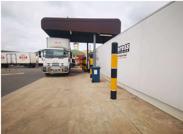
Plate 1: 64000 litre paraffin storage tanks and fuel filling station
