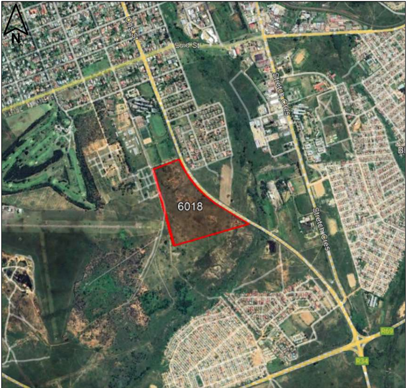
Figure 2-2: Aerial View, Site
