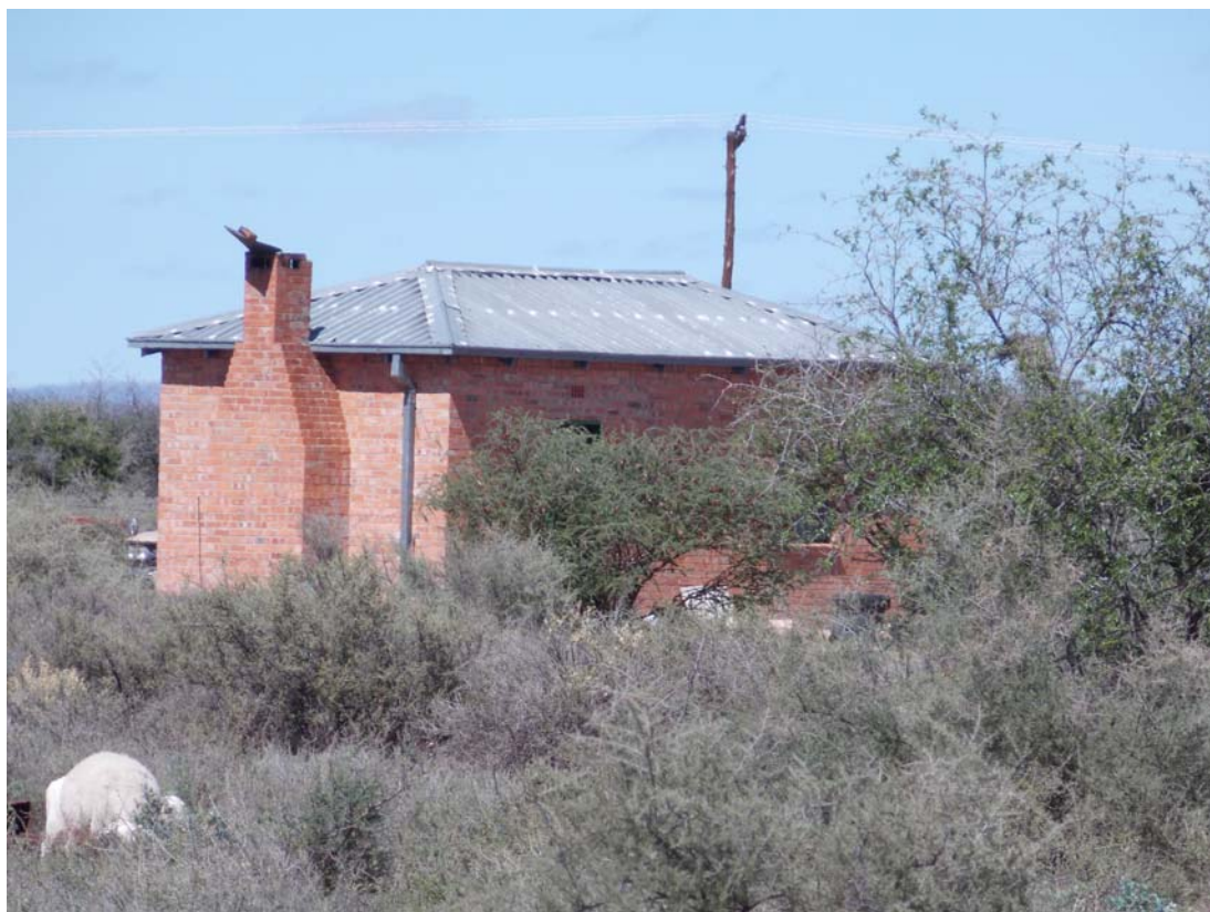
Figure 5.6: Labour housing on site
