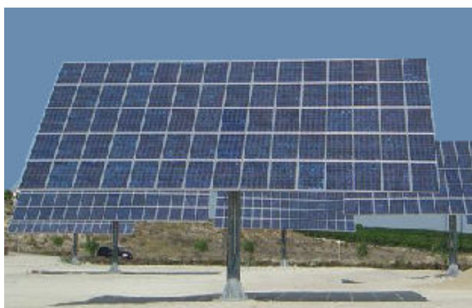
Figure 2.3: Illustration of a tracking photovoltaic panel
