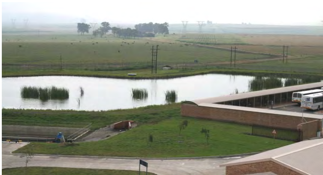
Figure 4.8.7.3(a): Storm Water PCD at Shaft Complex
