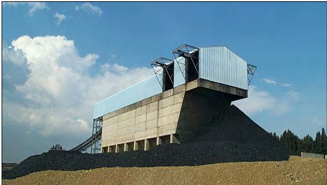
Figure 4.8.9.3.10(a): Surface ROM Coal Bunker, Throw-out and Emergency Stockpile
