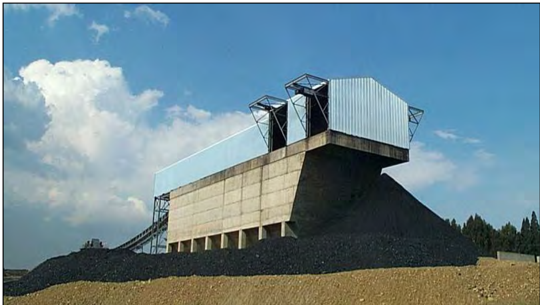
Figure 4.8.3(a): Typical Surface ROM Coal Bunker & Throw out
