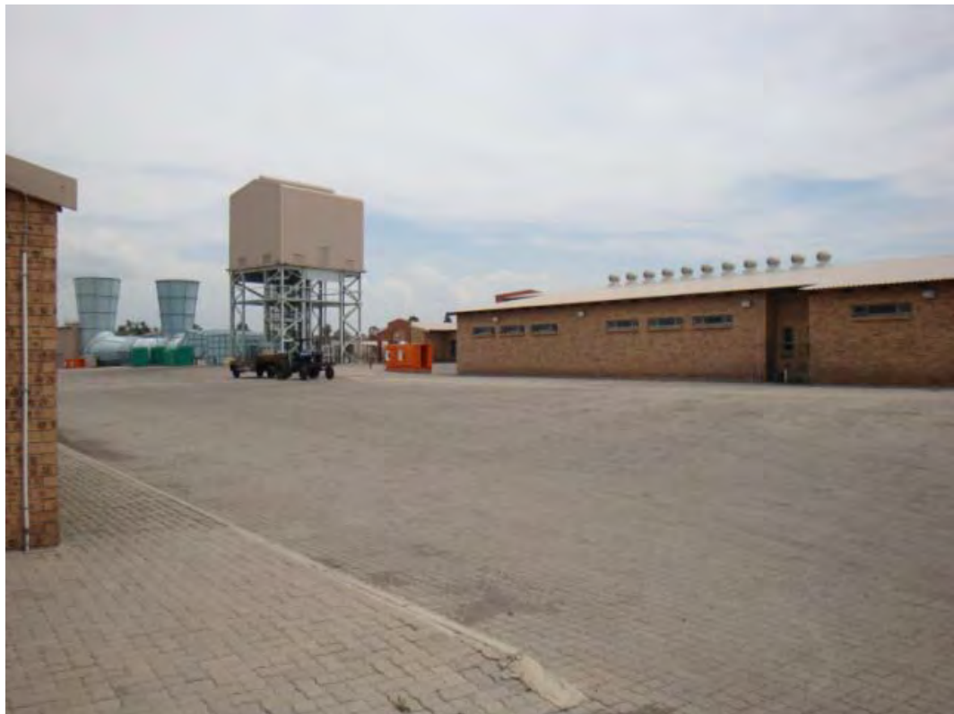
Figure 4.8.1.2.3(a): Paving to be used for Shondoni Internal Roads and Parking Areas
