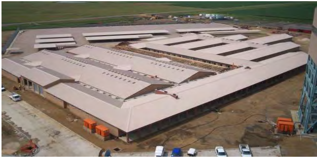
Figure 4.8.1.3(a): Office complex at Thubelisha
