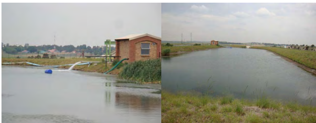
Figure 4.8.7.2(a): Service/Process Water Storage at iThemba lethu Shaft
