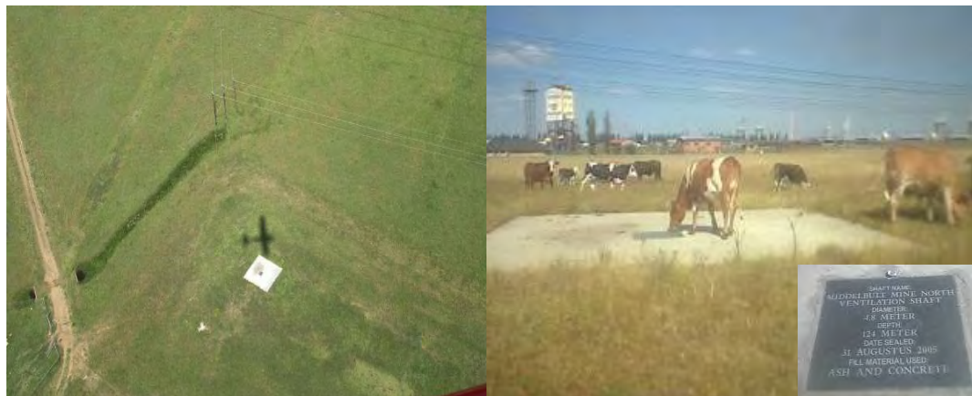
Figure 4.8.15(a): Typical Closed and Rehabilitated Vertical Shaft (Middelbult North Ventilation Shaft)
