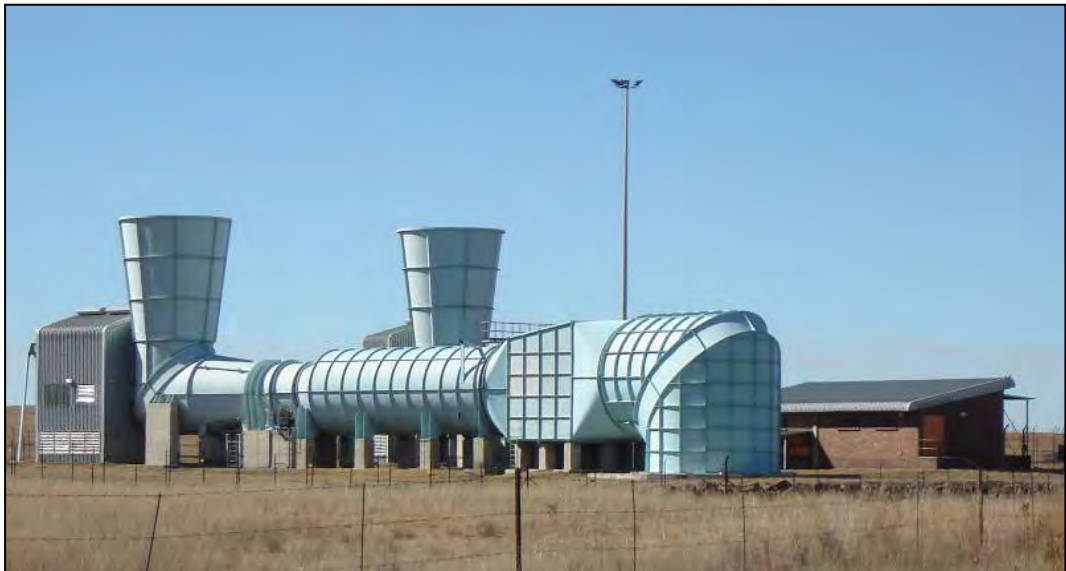
Figure 4.8.9.2.2(a): Typical Ventilation Shaft Surface Infrastructure
