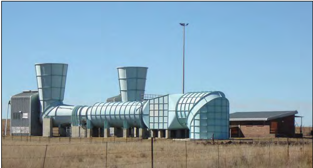
Figure 4.8.2.2(a): Typical Ventilation Shaft Surface Infrastructure
