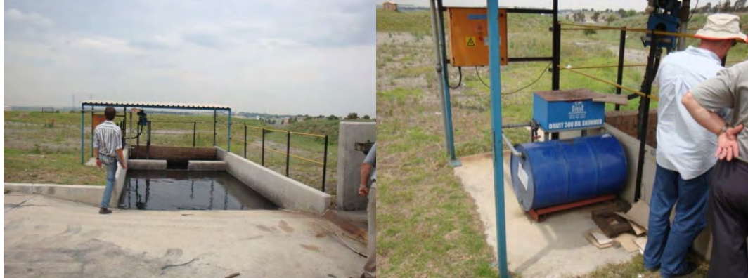
Figure 4.8.9.7.3(a): Typical Oil Trap and Skimmer System
