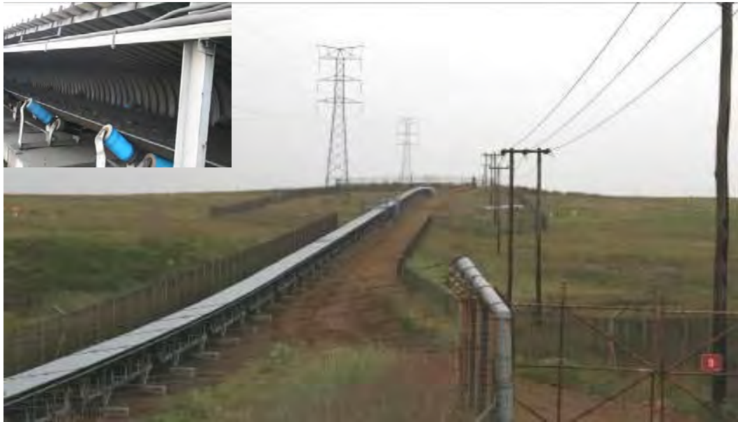
Figure 4.8.9.4.1(a): A Typical Overland Coal Conveyor
