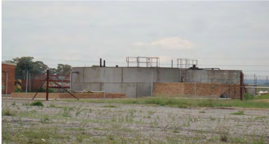
Figure 4.8.9.6.5(a): Typical Sewage Plant at Shaft Complex
