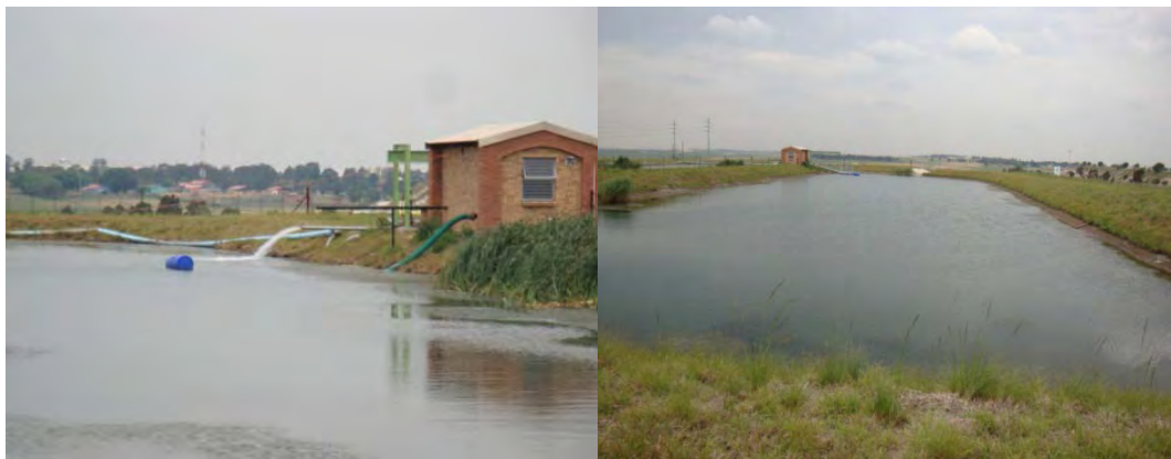
Figure 4.8.9.6.2(a): Service/Process Water Storage at Shaft Complex
