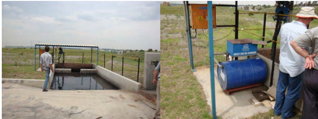
Figure 4.8.7.3(b): iThemba lethu Oil Trap and Skimmer System
