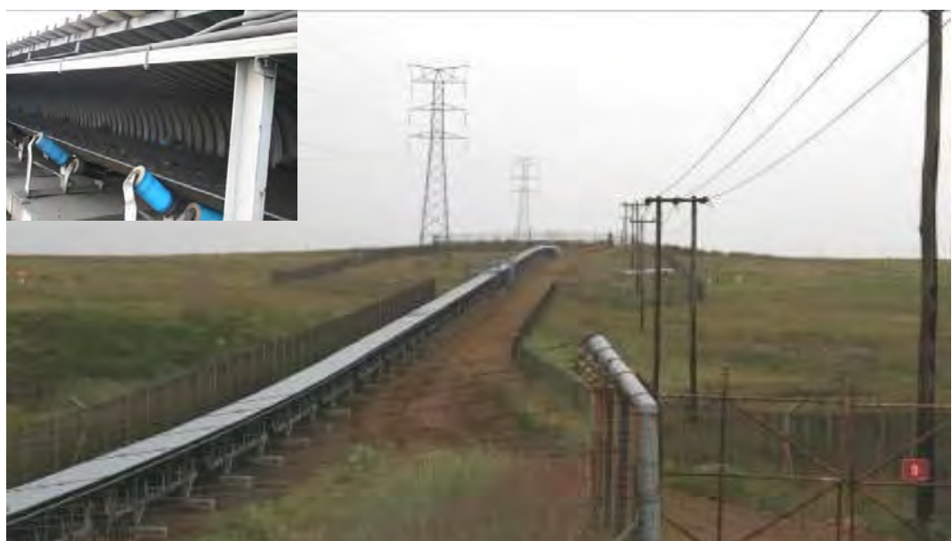
Figure 5.14.2.1(d): A Typical Overland Coal Conveyor
