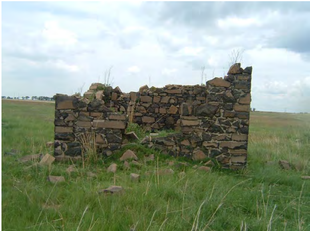
Figure 5.15.5.1(e): A possible 'bywonershuis' or a cool room ('koelkamer') on Witkleifontein 181IS which was constructed with dolerite stone in FC03
