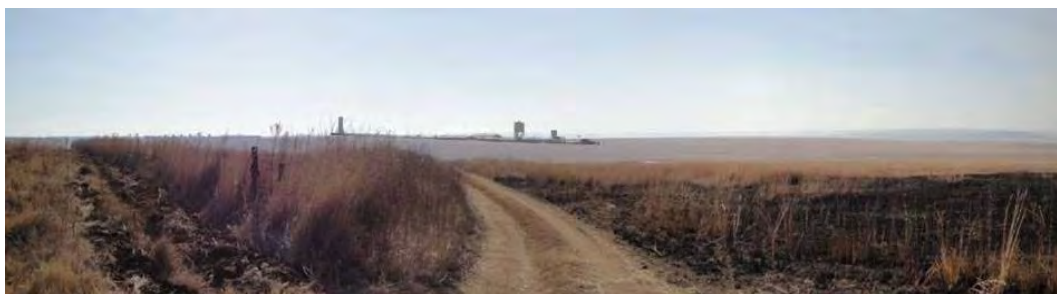
Figure 5.14.5.1 (b): Shondoni Shaft viewed from the West
