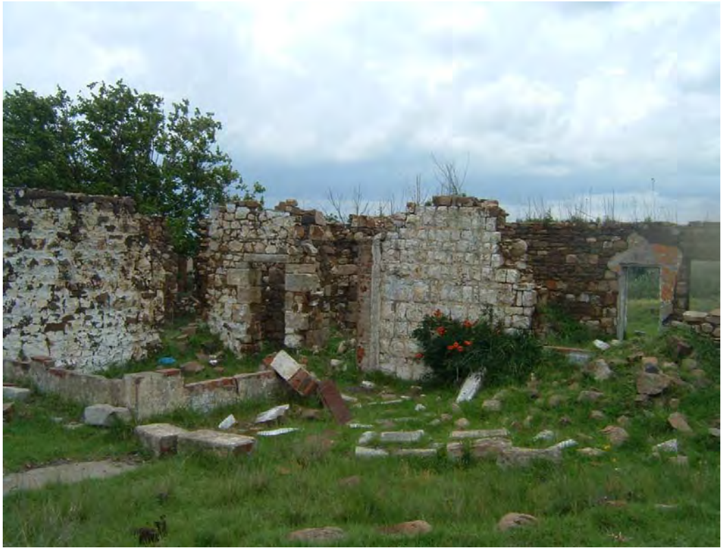
Figure 5.15.5.1(b): The main residence in FC01 on Kromdraai 128IS consists of a residence which was built with sandstone bricks and dolerite stone (above)
