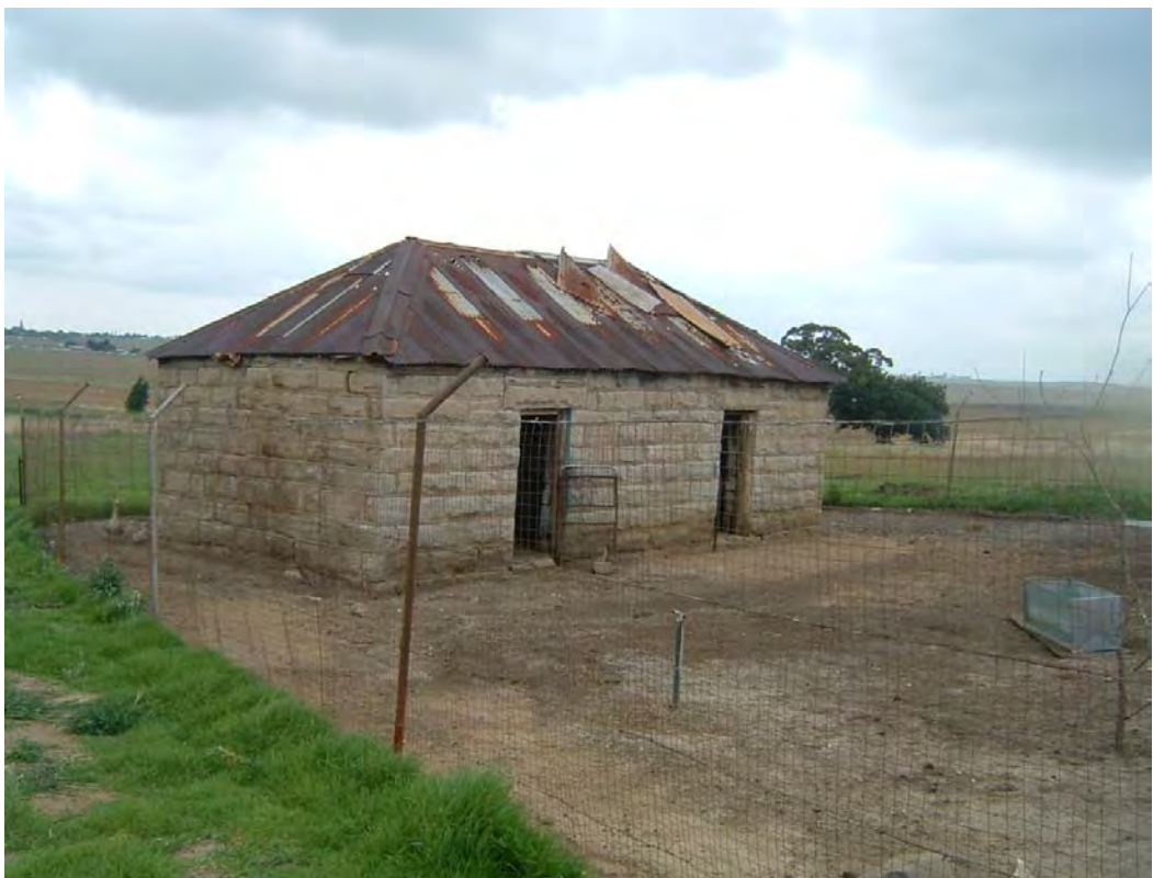
Figure 5.15.5.1(d): The “bywonerhuis” on Winkelhaak 139IS, also constructed with sandstone
