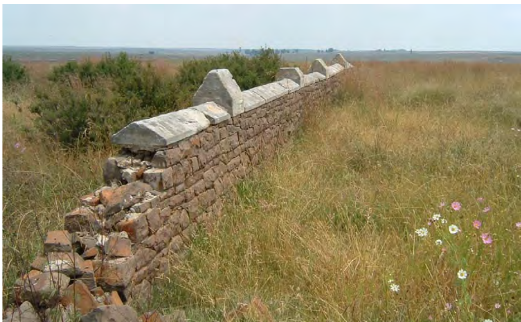
Figure 5.15.5.4(l): The wall that demarcates GY20 is constructed with dolerite stone and capped with sandstone trimmings
