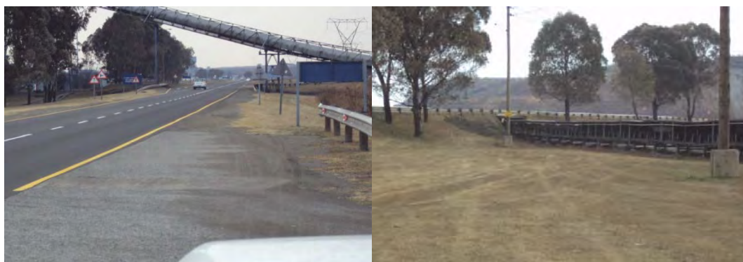
Figure 5.14.5.2(a): Examples of Conveyor Belts crossing over the Road versus under the Road
