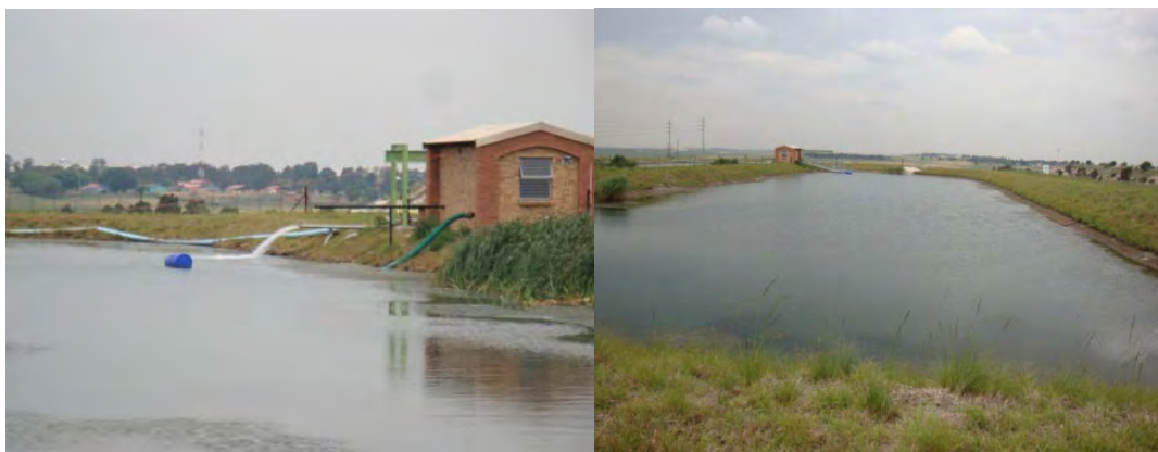
Figure 5.14.2.1(f): Service/Process Water Storage at Shaft Complex
