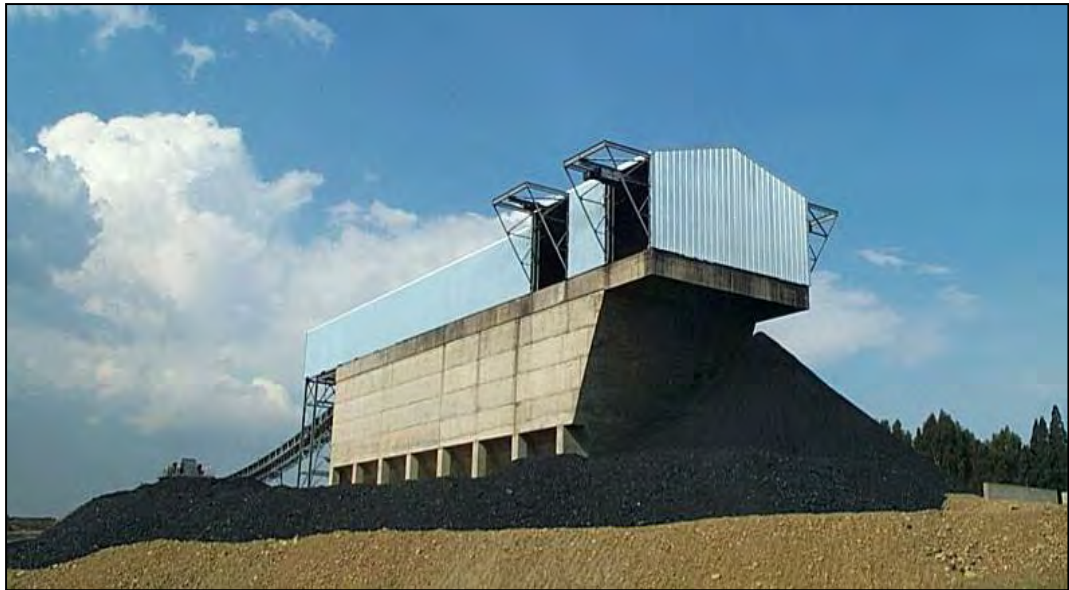
Figure 5.14.2.1(c): Surface ROM Coal Bunker & Emergency Throw-out
