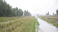
Vietnam - the left hand bank of the canal has been reshaped and stabilized with vetiver; the right bank has yet to be treated.
