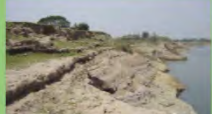
Cambodia - This very large bank on the Mekong River has been under continuous erosion. The land owner with assistance from TVNI is stabilizing using vetiver hedgerows.
