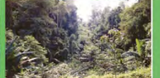
Thailand - a gas pipeline was laid through tropical forest. On steep slopes the right of way was stabilized with vetiver - native plants regenerated
