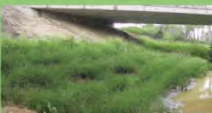
Australia - this river bank and bridge abutment have been stabilized with vetiver. Vetiver is an excellent interface for concrete and soil
