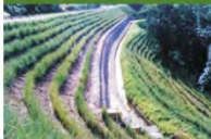
Malaysia - highway stabilization
