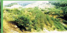
China - same fill less than a year later. After another two years this fill became fully forested. Untreated cut in background
