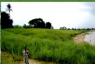
Cambodia - river bank stabilization
