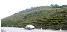
Vietnam - the Ho Chi Minh Highway has been stabilized with vetiver grass. The barriers and fills are stable and withstand cyclonic rainfall events
