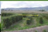
Australia - wastewater treatment
