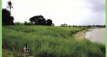
Cambodia - the bank in the previous image has been reshaped and planted with vetiver hedgerows. Very good growth seven months after planting.
