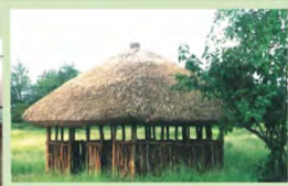
Zimbabwe - a nicely thatched meeting house using vetiver grass thatch. The thatch will last three times as many years due to its resistance to insects and fungus attack
