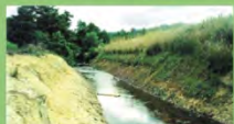
Australia - VS protects the right hand bank of a drain cut through acid sulphate soils of Queensland. Note left hand bank is devoid of any vegetation
