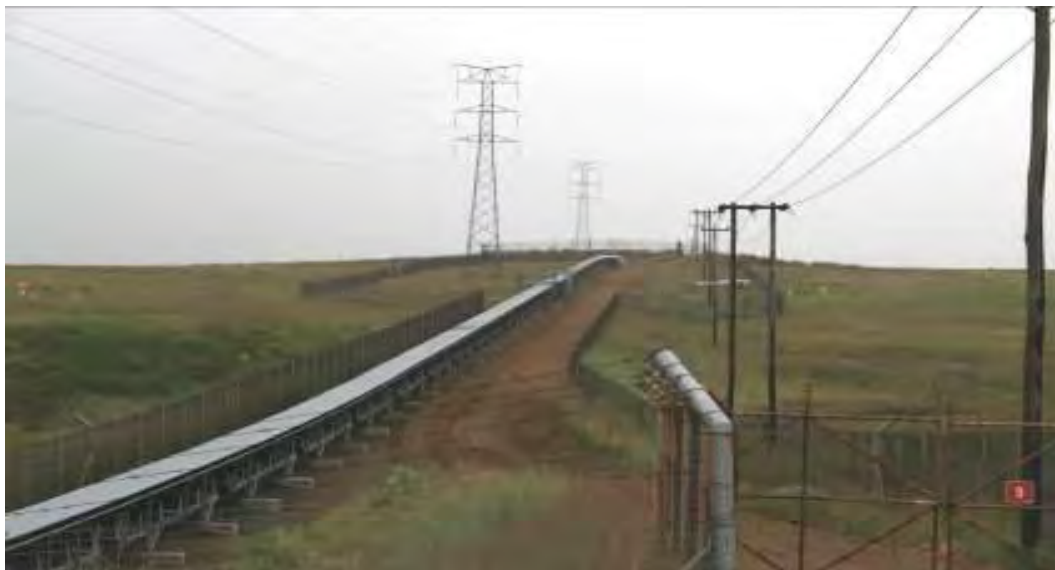
Figure 2.1(a): Typical Overland Conveyor with Associated Infrastructure
