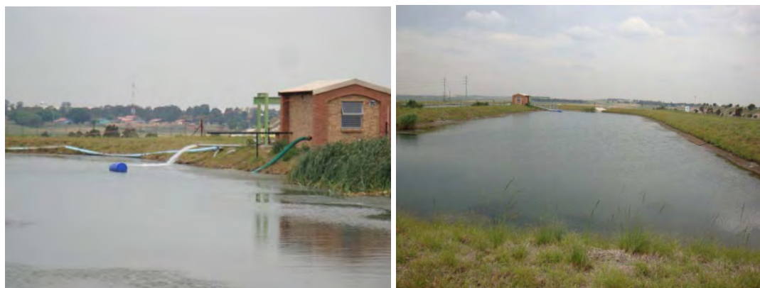
Figure 5.1(f): Service/Process Water Storage at Shaft Complex
