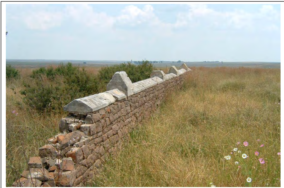
Figure 23- The wall that demarcates GY20 is constructed with dolerite stone and capped with sandstone trimmings (above).
