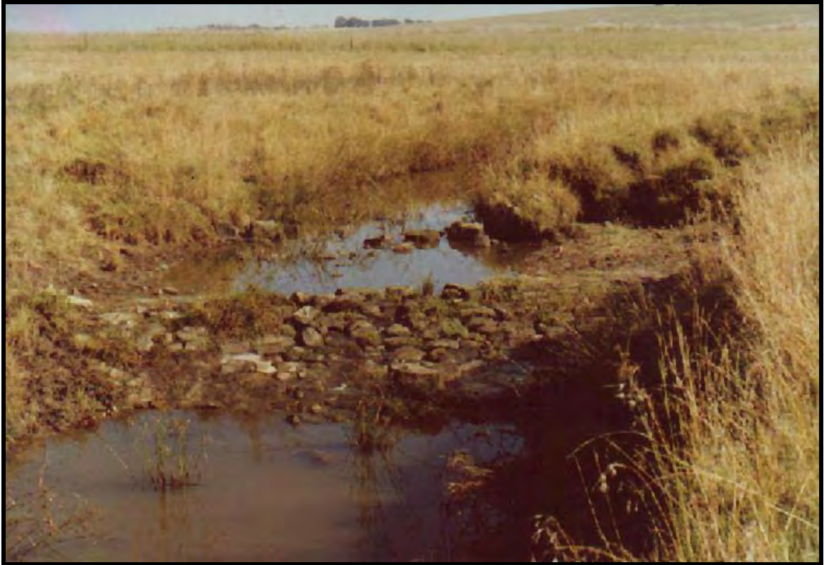
Figure 6. Kaalspruit downstream of the proposed development (Site 3), showing an artificial crossing that forms a riffle, and moderate erosion of banks.
