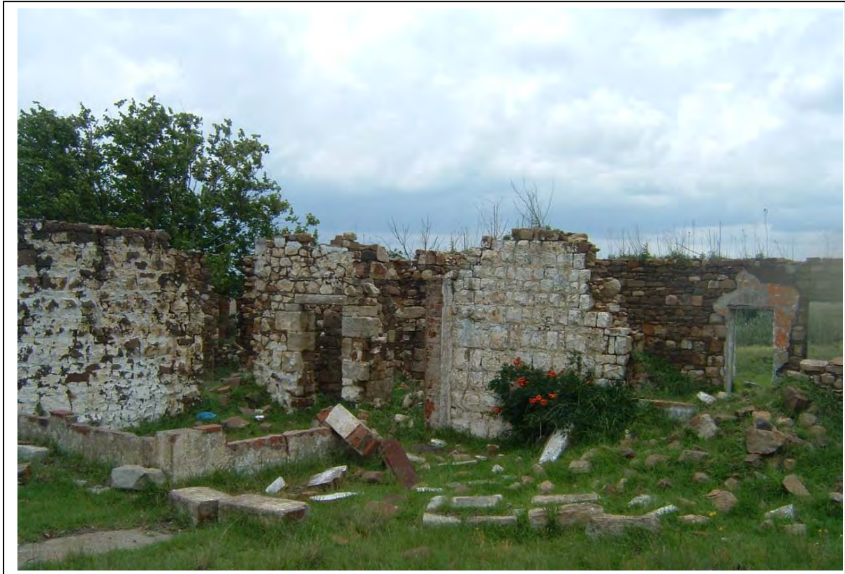
Figure 4- The main residence in FC01 on Kromdraai 128IS consists of a residence which was built with sandstone bricks and dolerite stone (above).
