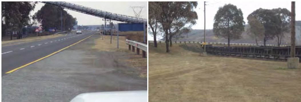
Figure 7.2(a): Examples of Conveyor Belts crossing over the Road versus under the Road
