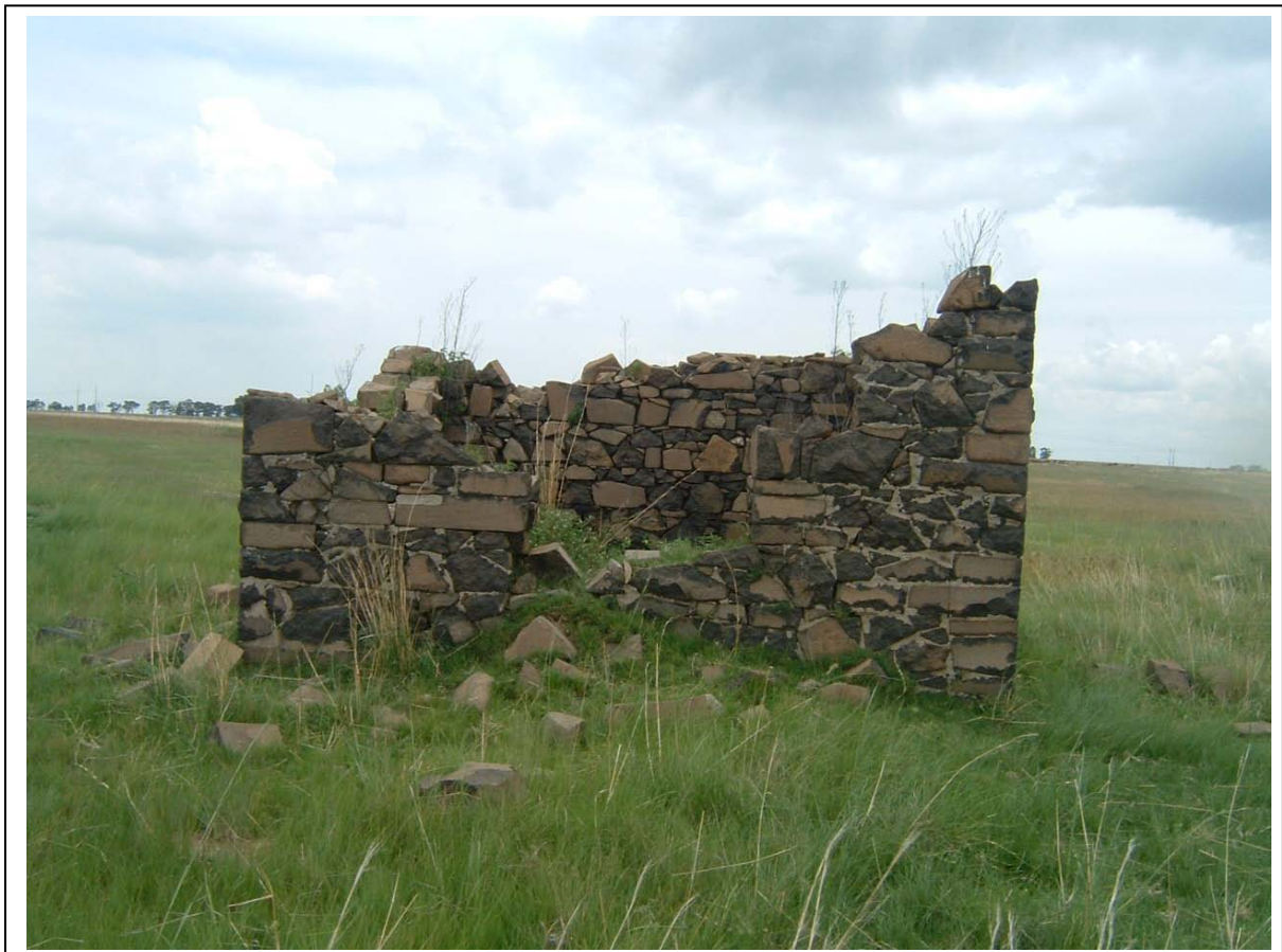
Figure 7- A possible 'bywonershuis' or a cool room ('koelkamer') on Witkleifontein 181IS which was constructed with dolerite stone in FC03 (above).
