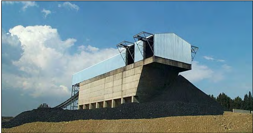
Figure 5.1(c): Surface ROM Coal Bunker & Emergency Throw-out
