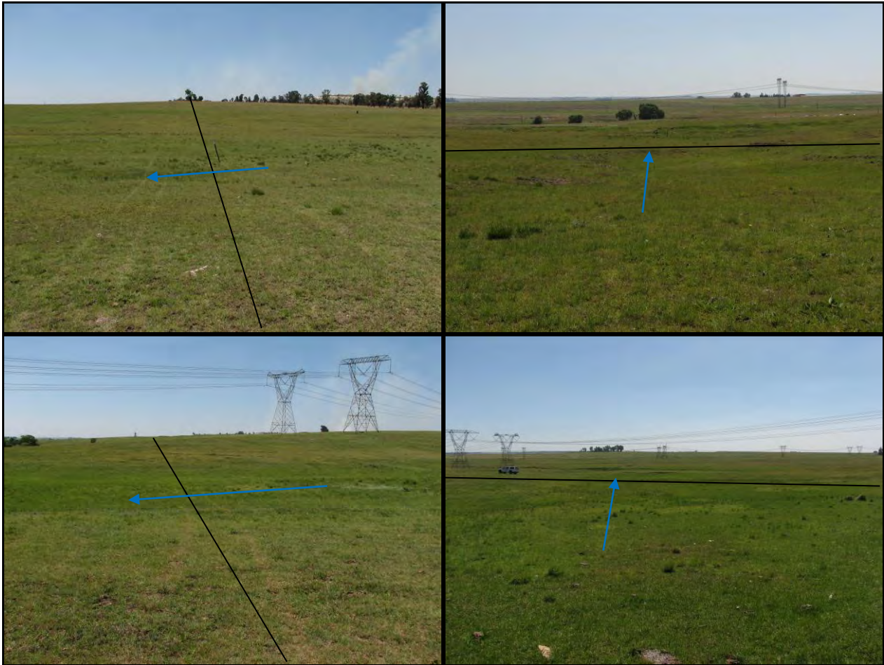
Figure 29. Photographs of crossing 6 and 7 along the conveyor route. Black line indicates approximate conveyor route and blue indicates flow direction.
