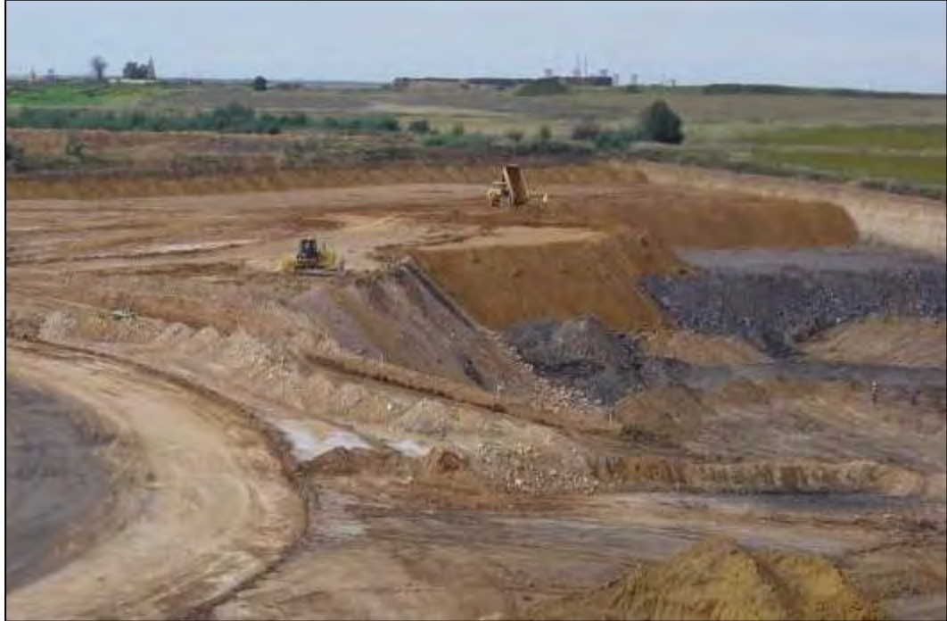
Figure 3.1.7.9 (a): Rehabilitation taking place on mined-out Blocks
