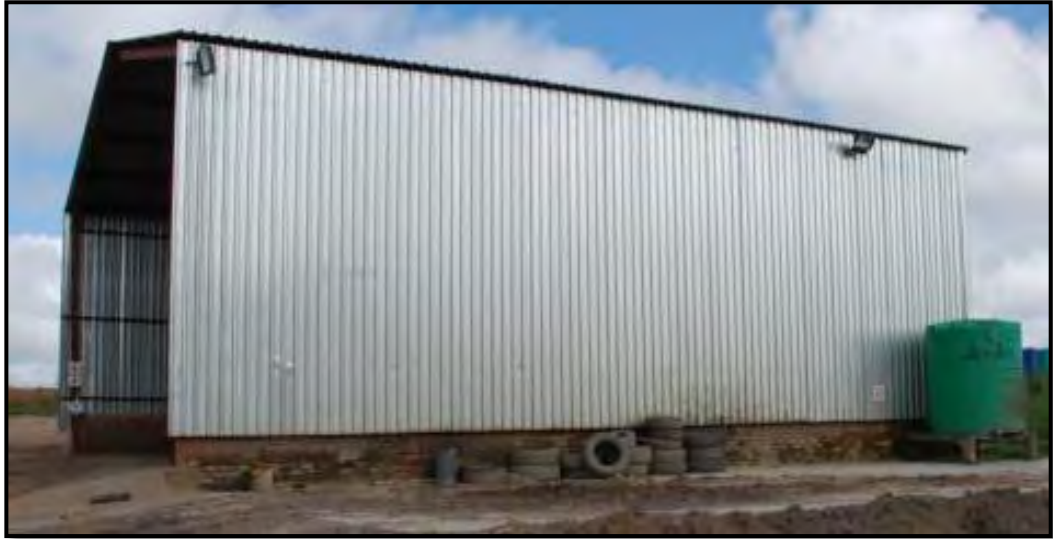
Figure 2.19.4.2 (a): Typical Work Shop in the Contractor's Yard.
