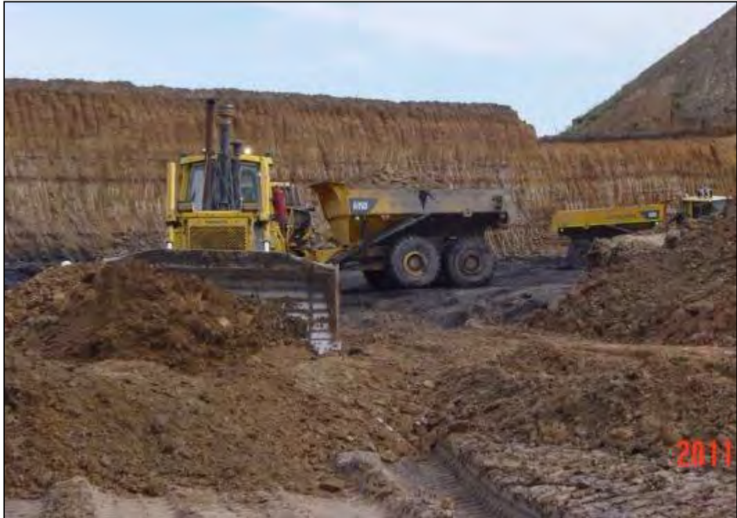
Figure 3.1.7.4 (a): Dozing of Overburden towards the Spoils
