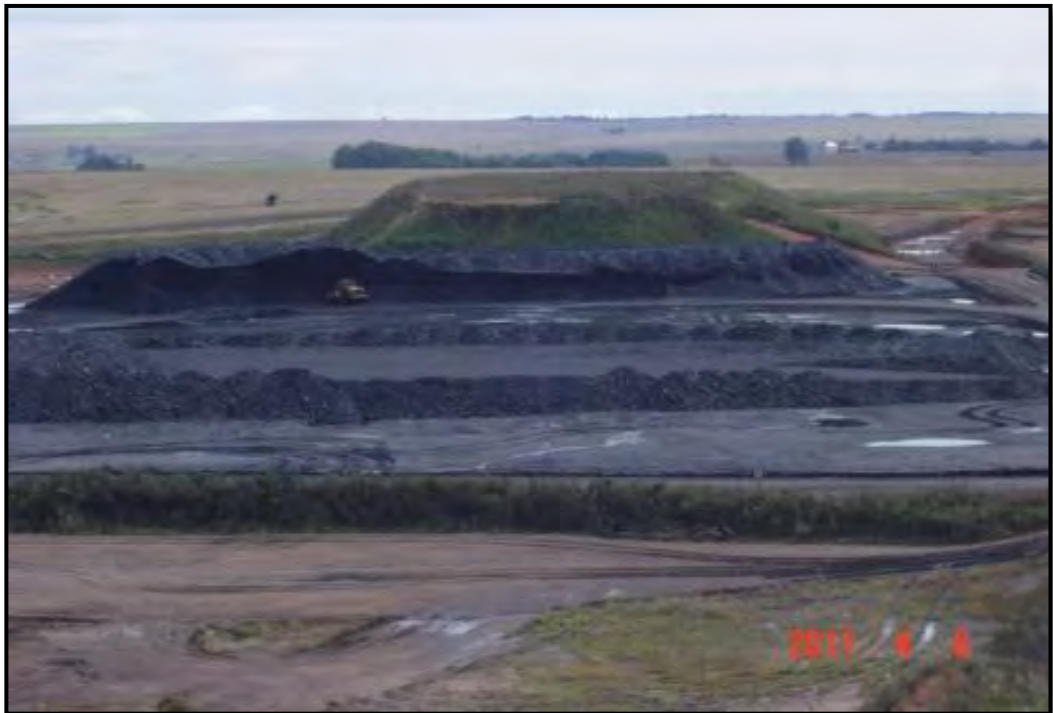
Figure 2.19.4.2 (b): Typical ROM Stockpile.
