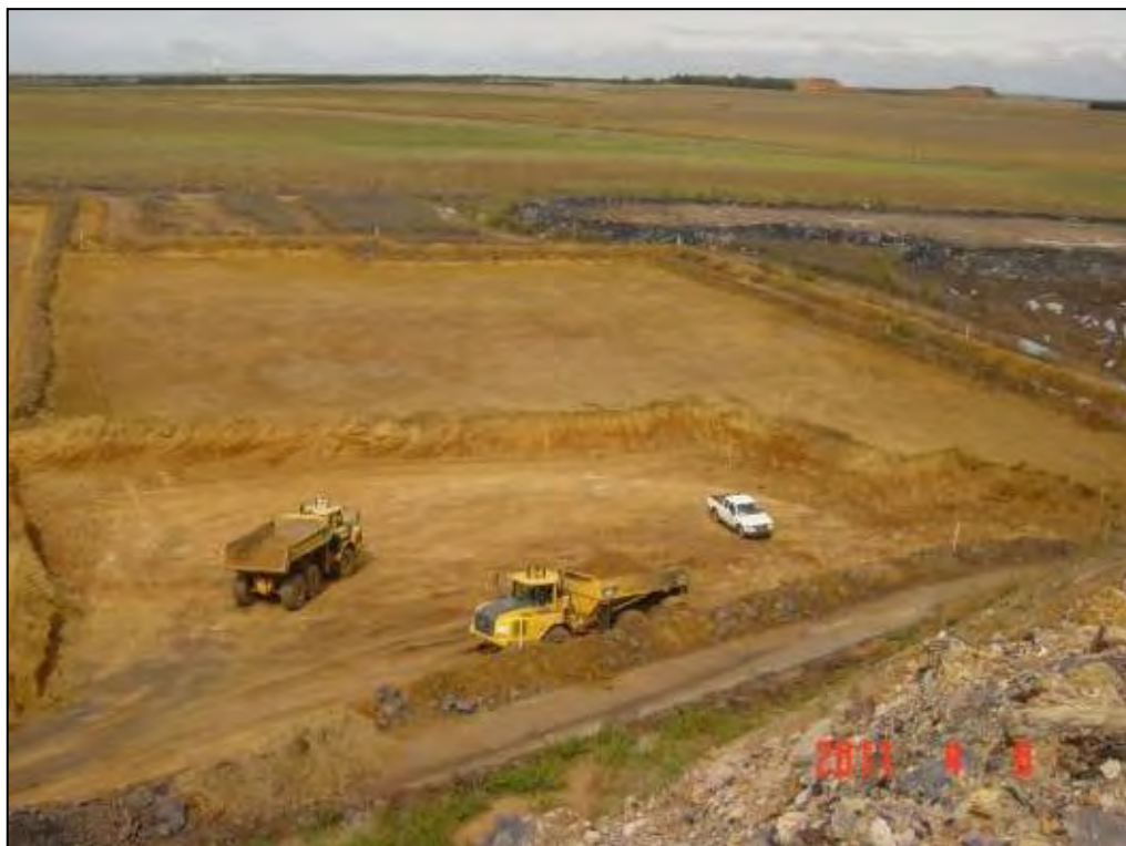
Figure 3.1.7.2 (b): Removal of Softs within demarcated Block
