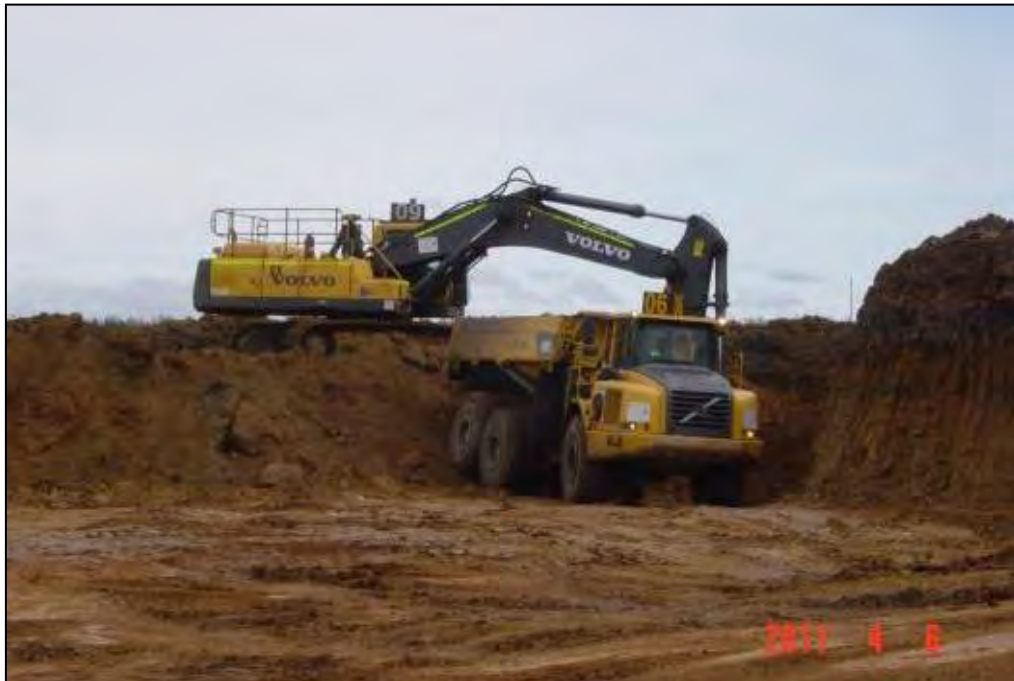
Figure 3.1.7.2 (a): Removal of Soft Overburden (Softs) using an Excavator and ADT
