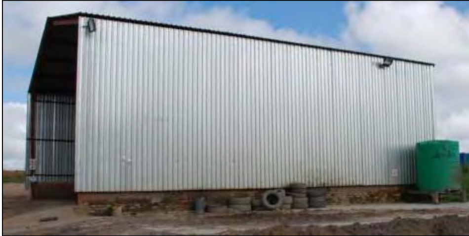
Figure 3.1.5.2.6 (a): Typical Work Shop in the Contractor's Yard.
