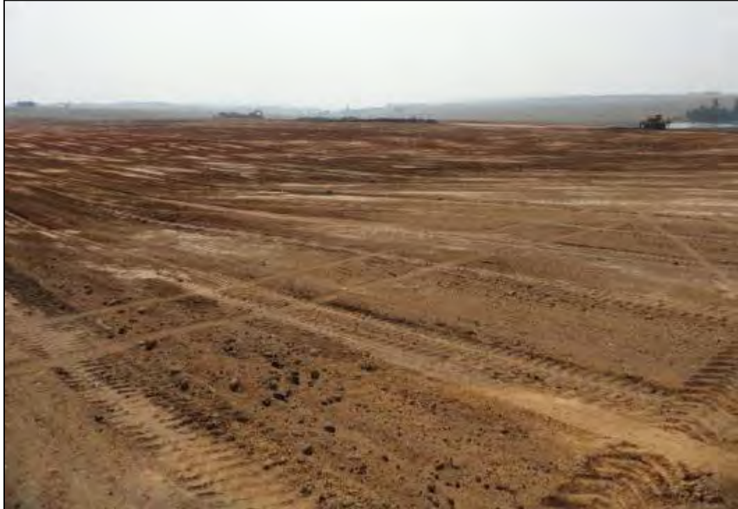
Figure 3.1.7.9 (b): Free Draining Rehabilitated Area. Topsoil is ready to be Re-vegetated
