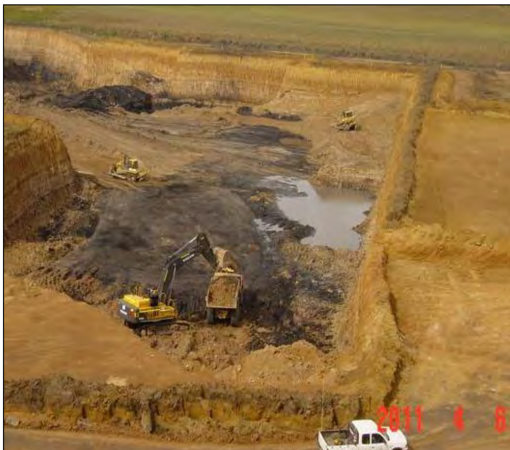
Figure 3.1.7.5 (b): Removal and Dozing of Hard Overburden within designated Block
