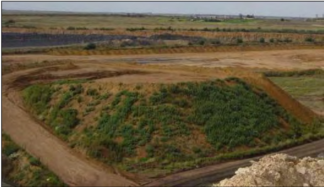
Figure 3.1.5.7 (a): Typical re-vegetated Soil Stockpile.
