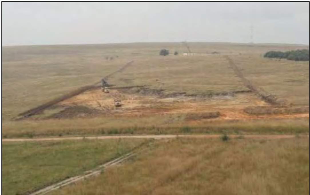
Figure 3.1.7.1 (a): Removal of Topsoil within demarcated Block
