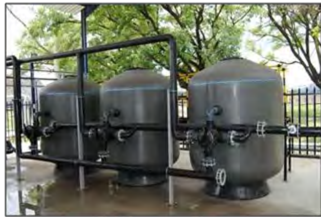
Figure 3.1.5.17.4 (b): Manganese Dioxide Filters
