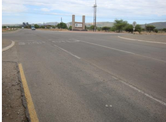
AP-10) D1813 Rd/ Access Road Intersection
