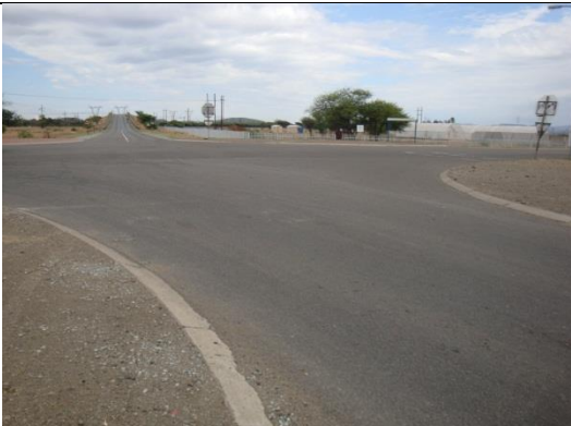
AP-10) D1813 Rd/ Access Road Intersection
