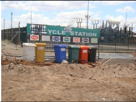
Recycle Station – Slag and Stockpiles
