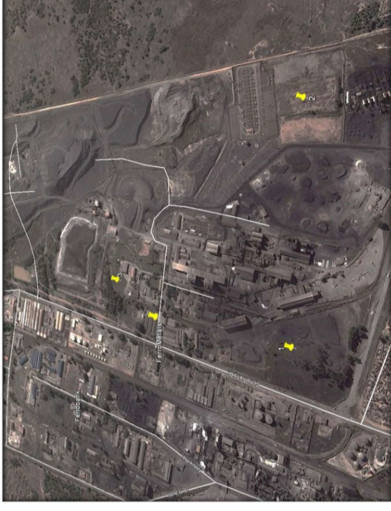
Figure 2(a): Aerial photograph of the Ferrometals Site indicating the three historical slimes dams footprints.
