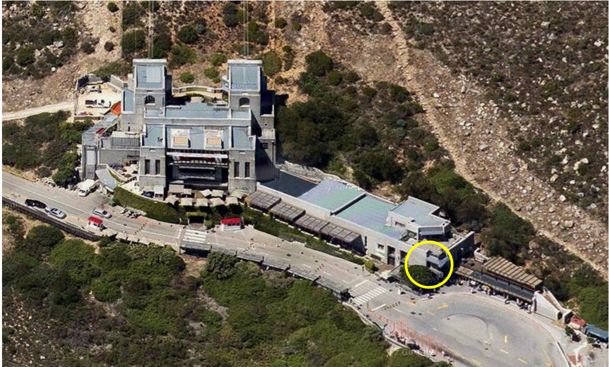
2016 oblique aerial photo of Lower Station from the north, with the location of the proposed alterations circled in yellow. (Source: Google)
