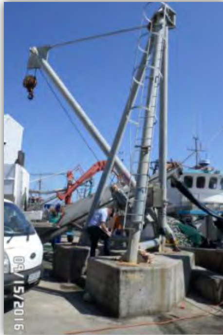
Figure 1.2.3.1c: Structural cracks to be repaired
