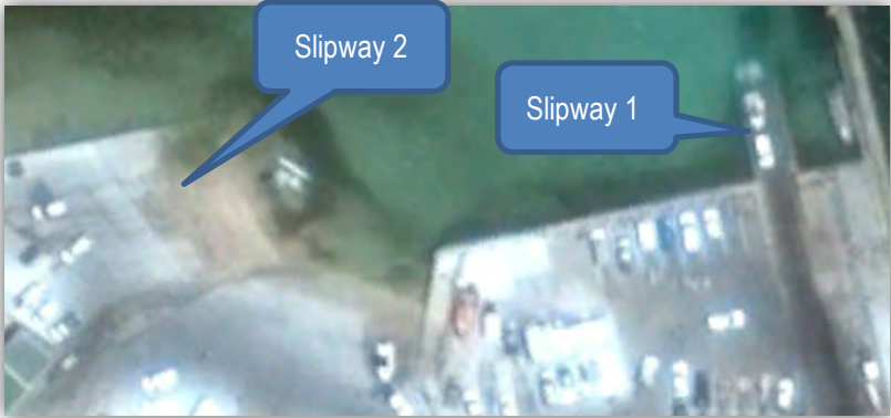
Figure 1.2.4.1: Locality of Slipways 1 and 2.
