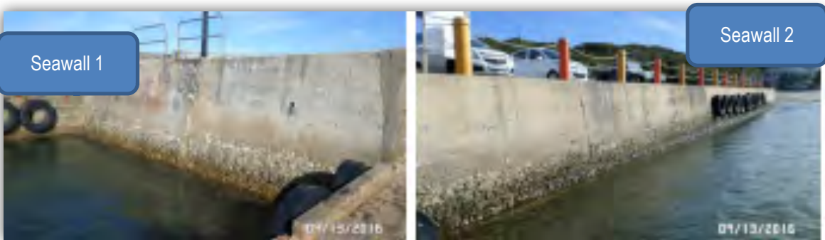
Figure 1.2.3.1b: Views of Seawalls 1 and 2
