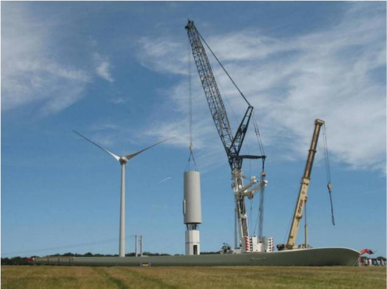
Plate 2-4: Assembly and erection of the tower sections using cranes
