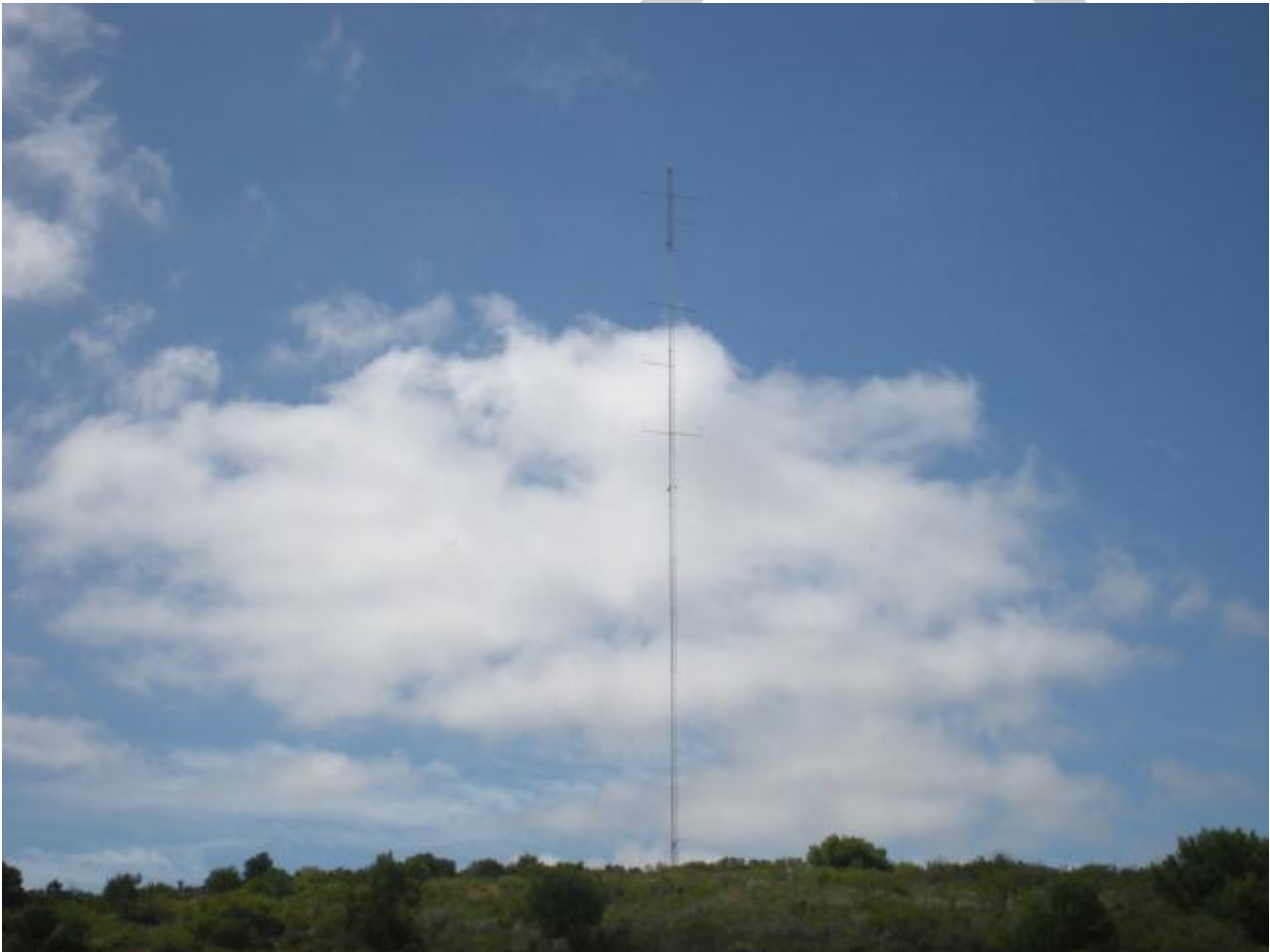
Plate 2-2: An example of a meteorological mast
