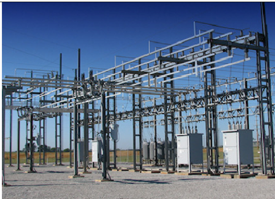
Figure 3: Illustration of a 132kV Distribution Substation
