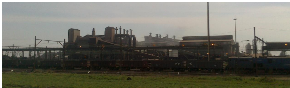
Figure 2.2: View of Transalloys smelter complex taken from the south west
