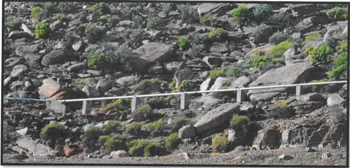
Photo 2: Typical aboveground construction method for the pipeline
