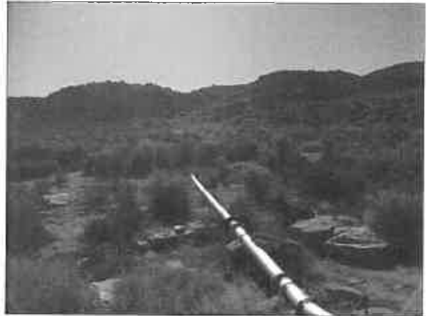
Figure 33. Alternative A4. Existing pipeline from Carolusberg to Okiep. View facing north
