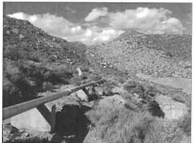
Figure 35. Alternative A4. Existing pipeline from Okiep to Carolusberg. View facing south
