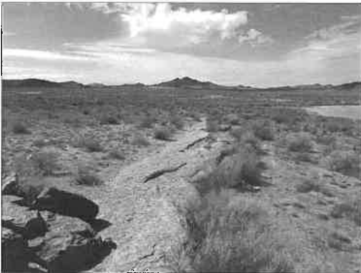
Figure 13. Alternative A1 (the preferred route). View facing east to the Concordia/Carolusberg road. Thereafter, the route will be aligned directly alongside the gravel road to Carolusberg
