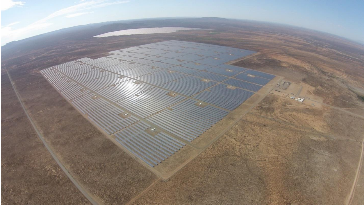
Figure 2: Photo showing the aerial view of the PV facility
