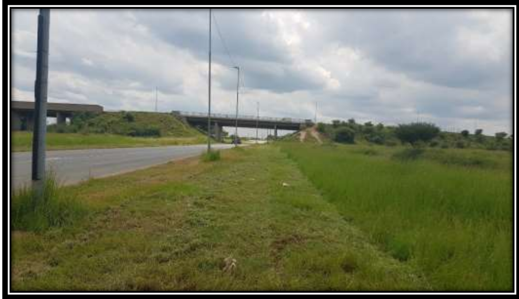
Photograph 1: The R49 Road (Mmabatho - Zeerust Road), also referred to as Shippard Street borders the site to the north.
