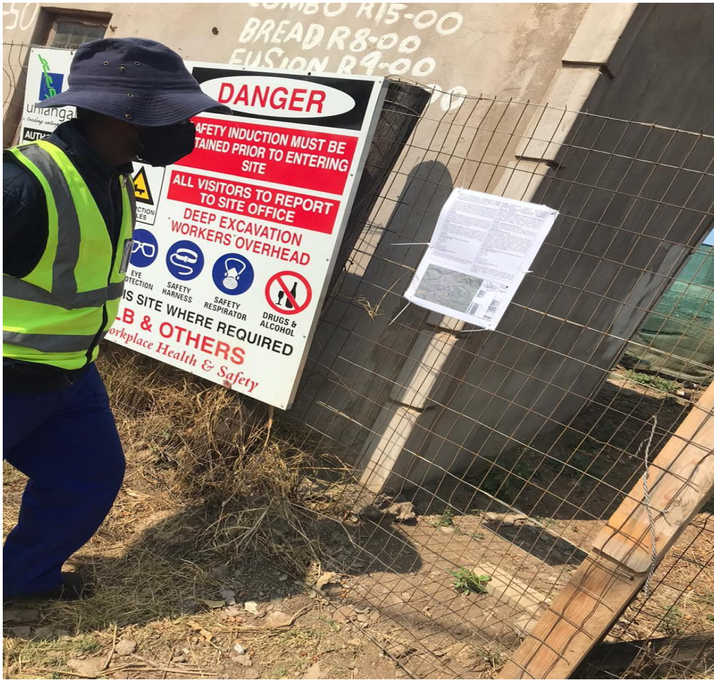
Site Notice 1 – Current Phase 1 Construction Camp Site
