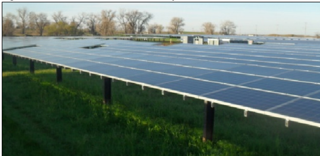
Figure 8 Frontal views of the PV arrays mounted on horizontal 1-axis tracker
