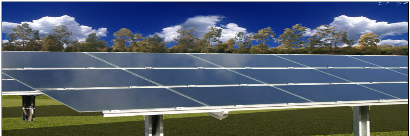
Figure 6 Frontal view of PV arrays mounted on fixed mounting systems
