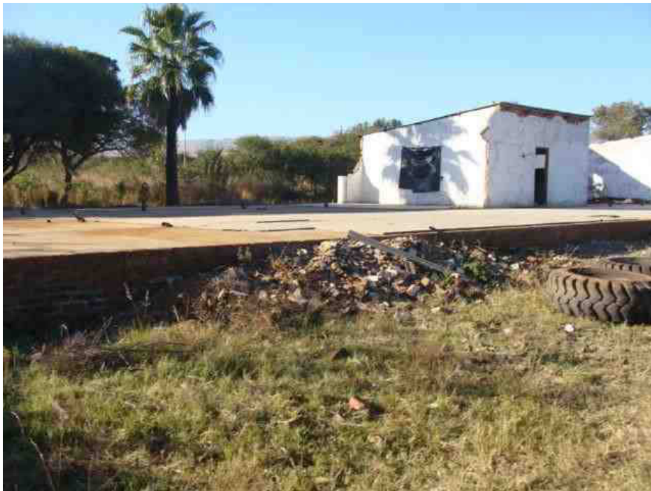
Figure 6: Farm infrastructure in ruins inside of the surveyed area.
