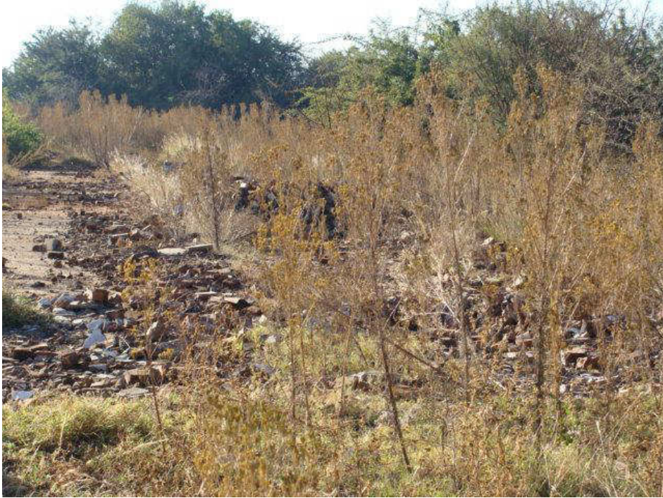
Figure 5: View of one of many concrete floors found in the surveyed area.
