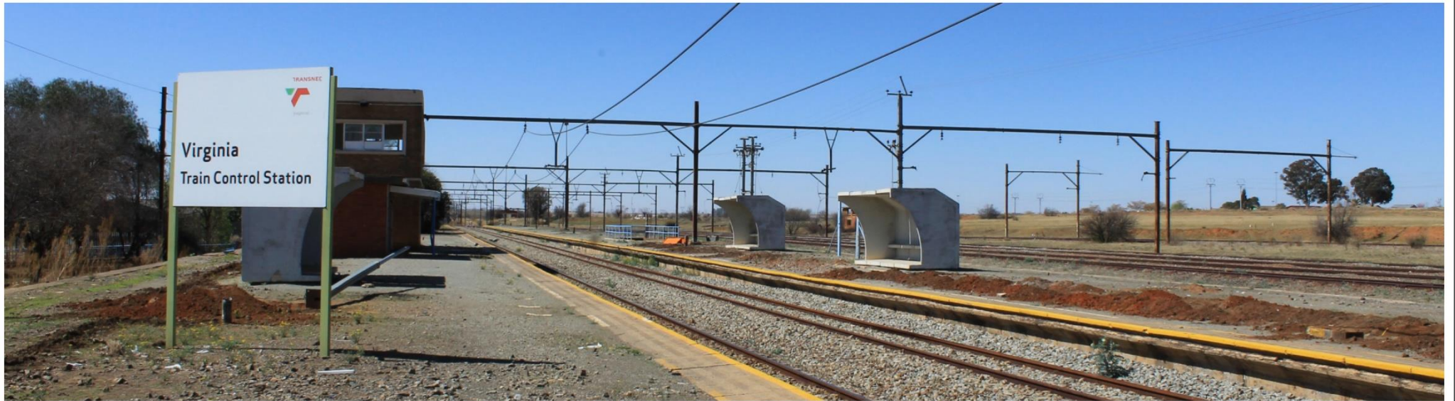
CL 21 along road from N1 to Virginia, Virginia Train Control Station.
