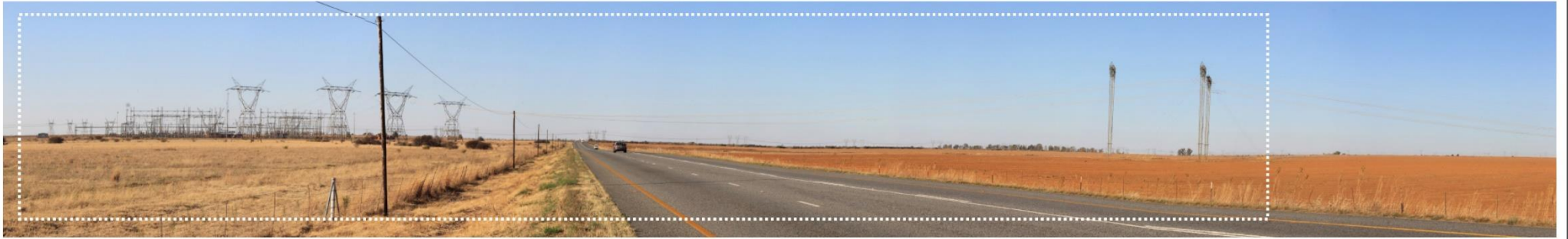
CL 40 Virginia Power Line
