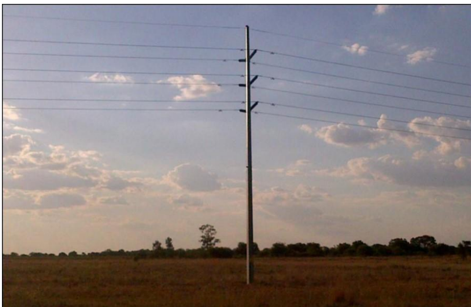
Figure 7. Steel monopole structure for a 132 kV powerline (double-circuit)
