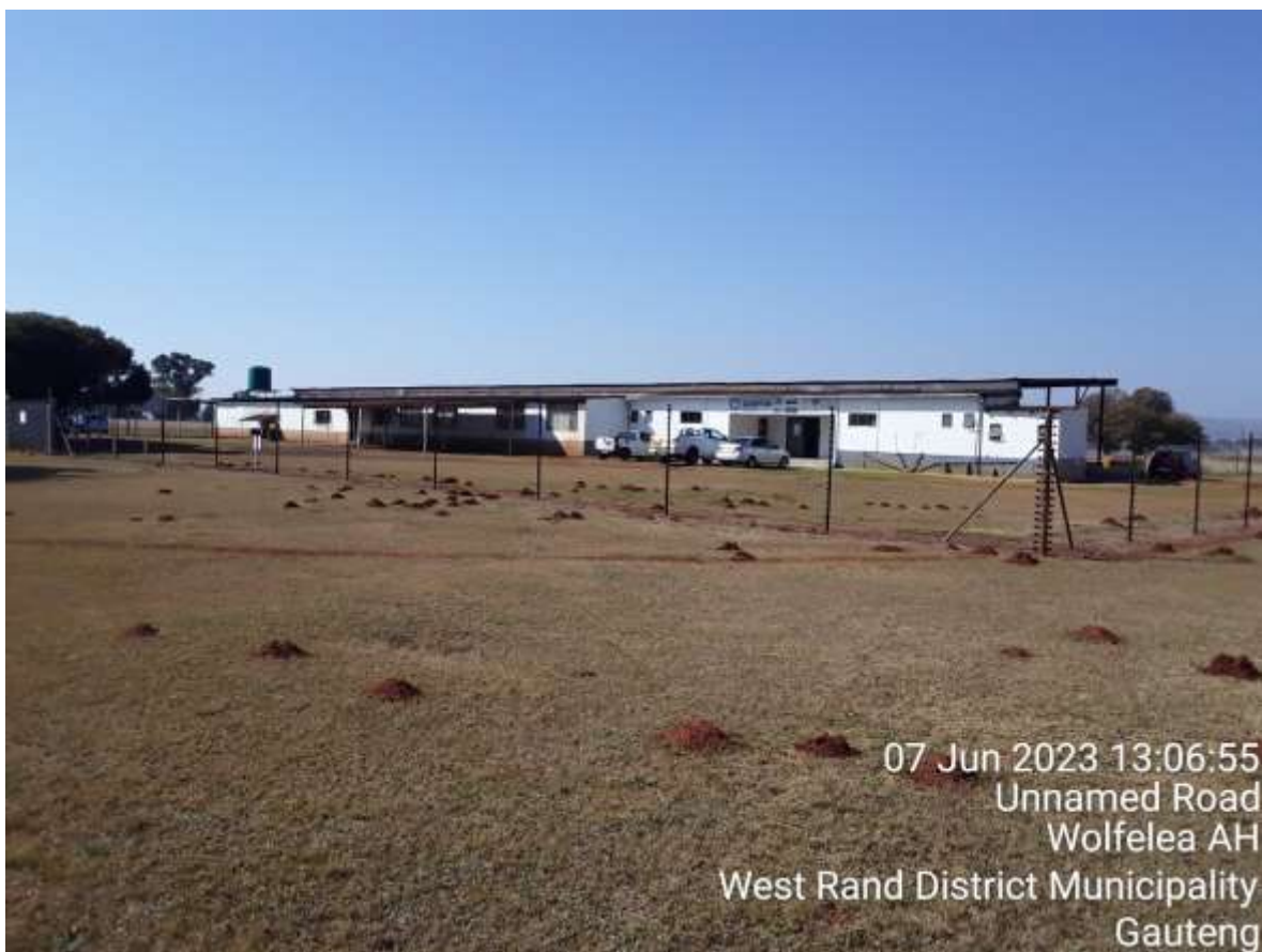
Northeast photo of the project site
