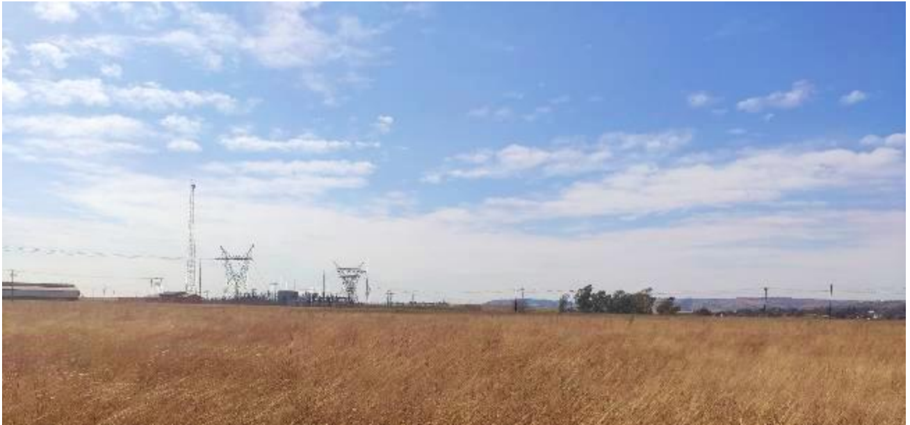
Figure 3: Overhead powerlines in the Development Area.
