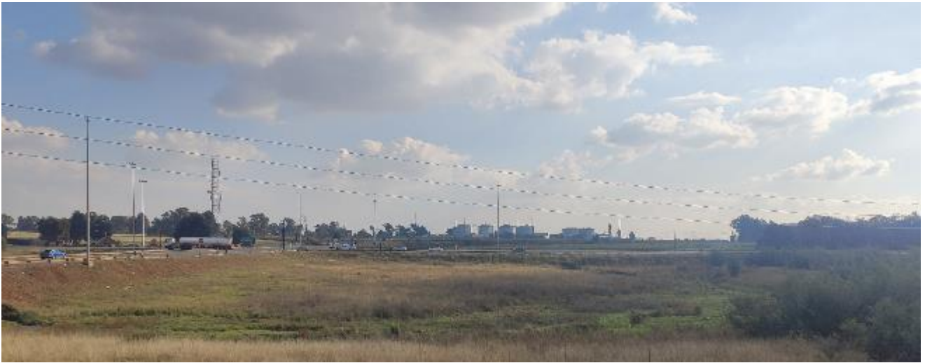
Figure 3: Overhead powerlines in the Development Area.
