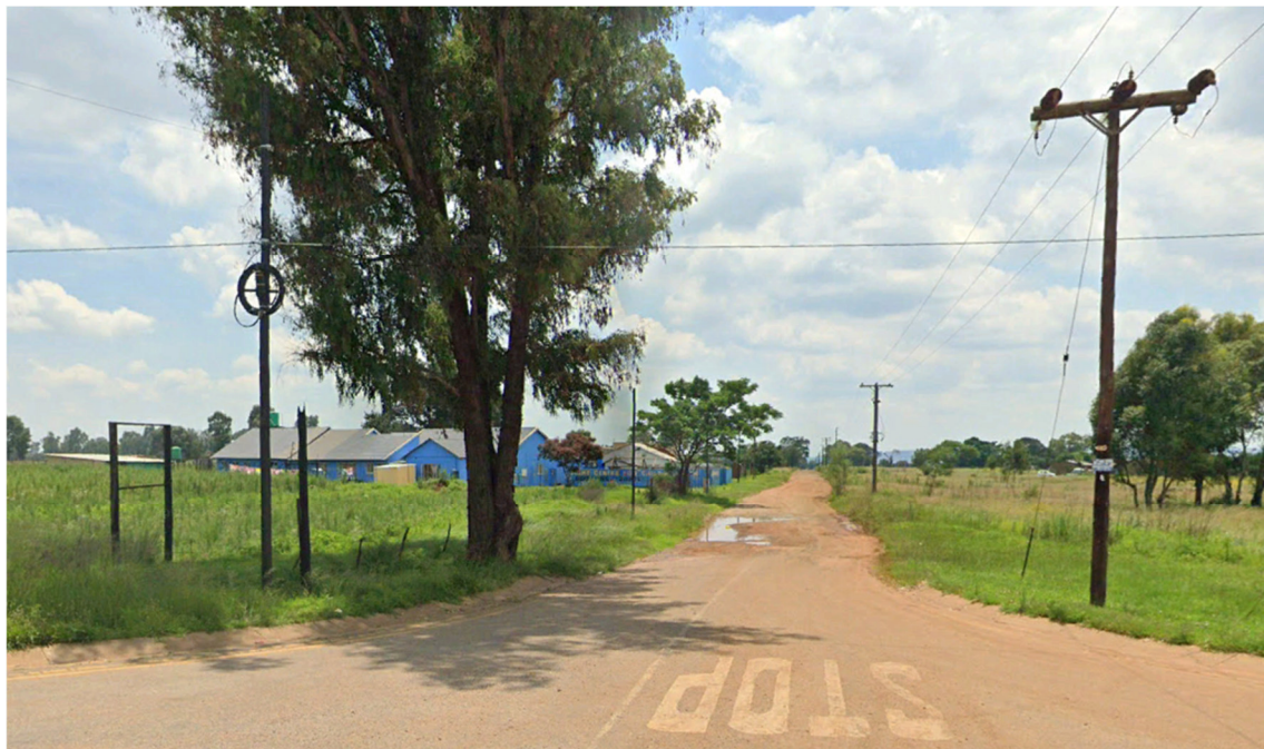
Figure 4-3: Existing farm road towards site from R24
