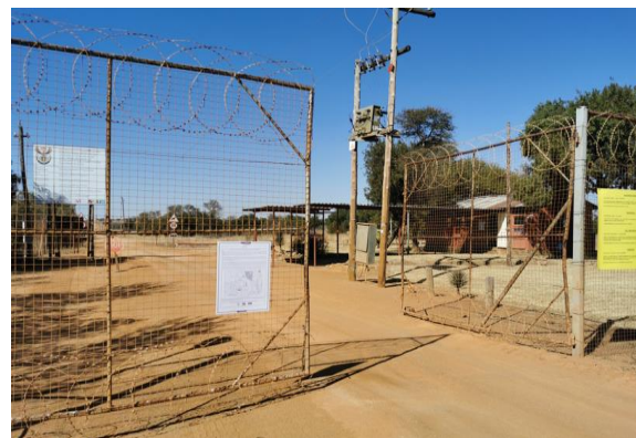
Figure 5: Security access point for the SAPS training facility
