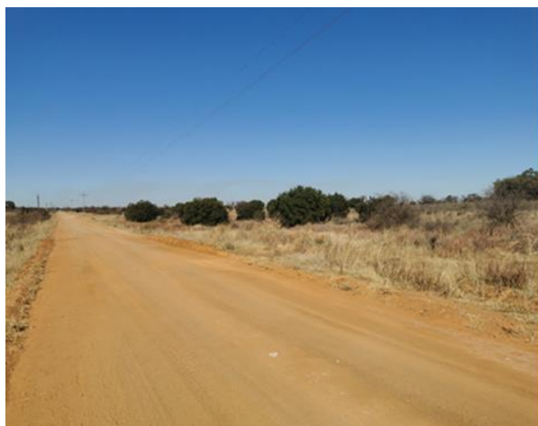
Figure 6: The existing access road currently being used on site
