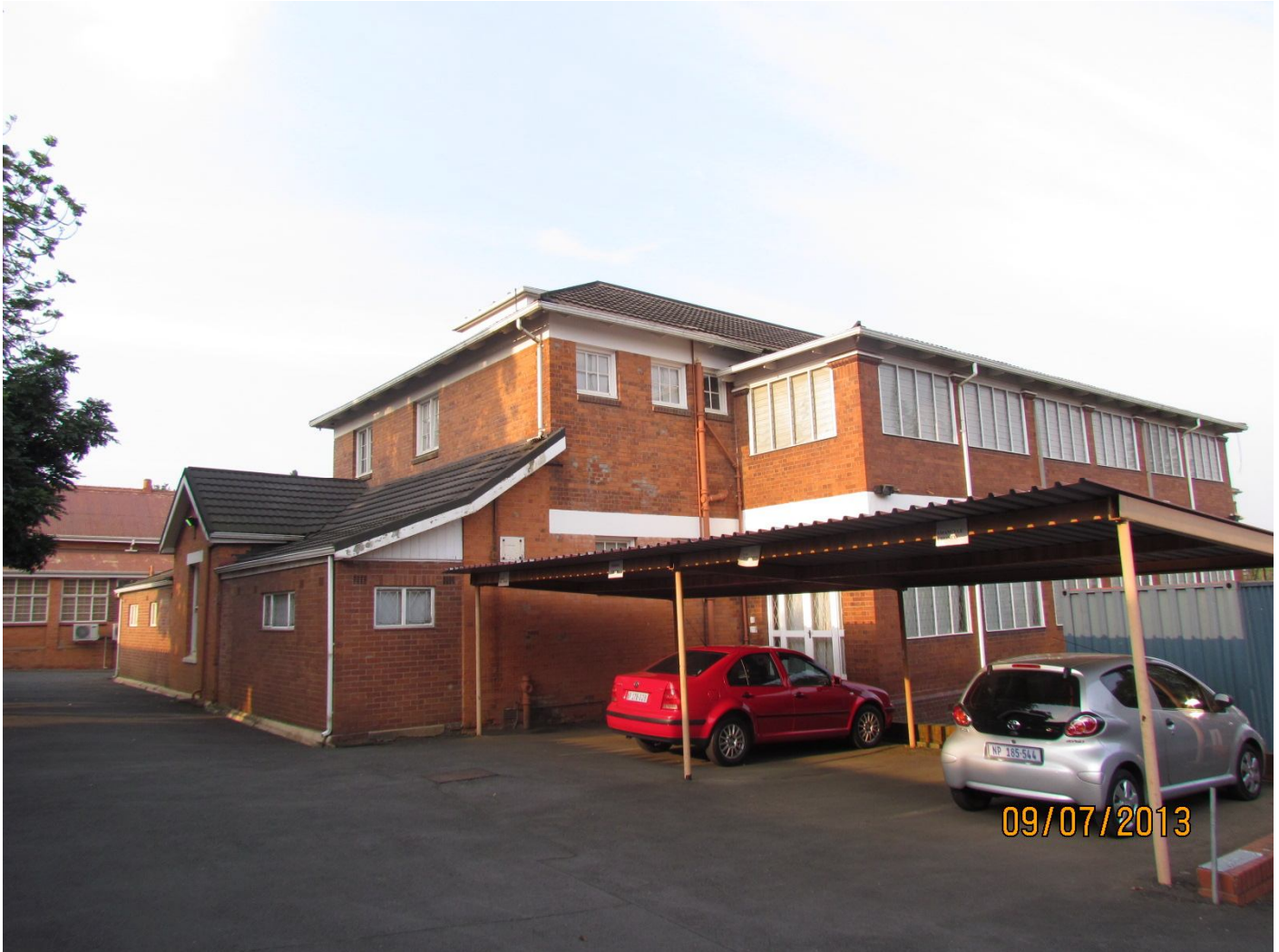
View looking East
