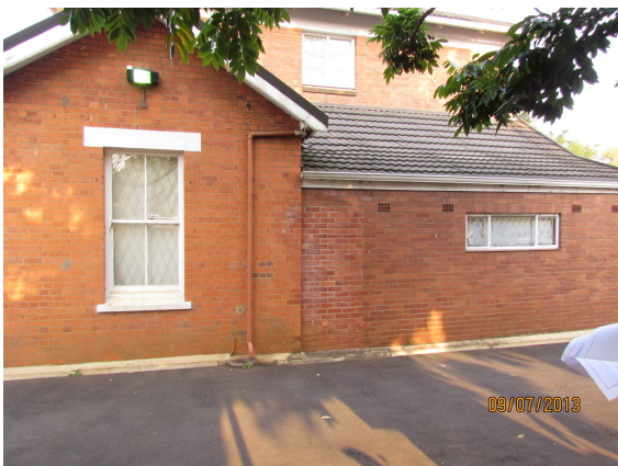
View looking South East
