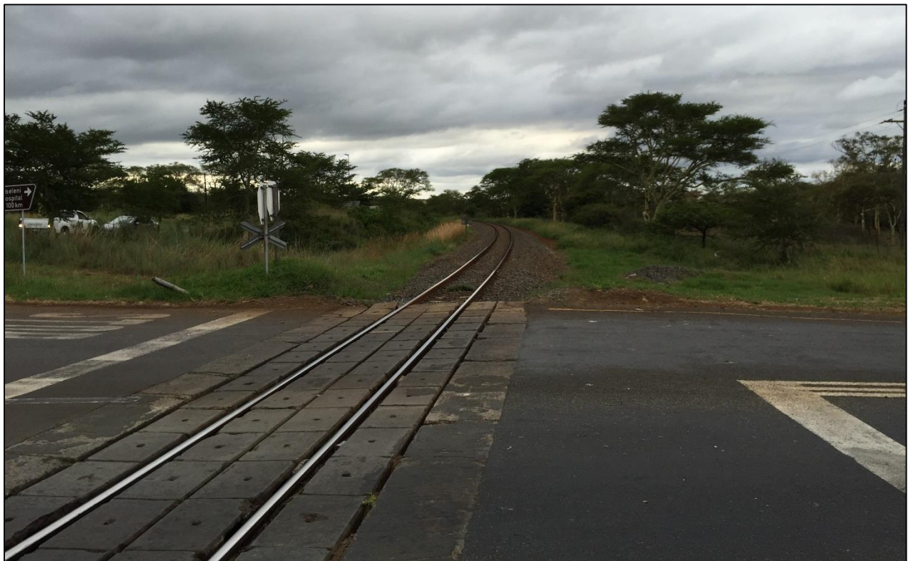
Plate 2. The railway line over which a bridge is proposed, to provide safe crossing for vehicular and foot traffic.
