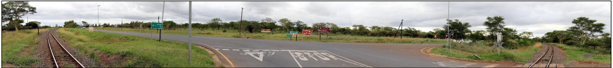
Plate 7. A panoramic view, from the east, of the R22 intersection with the railway mainline.
